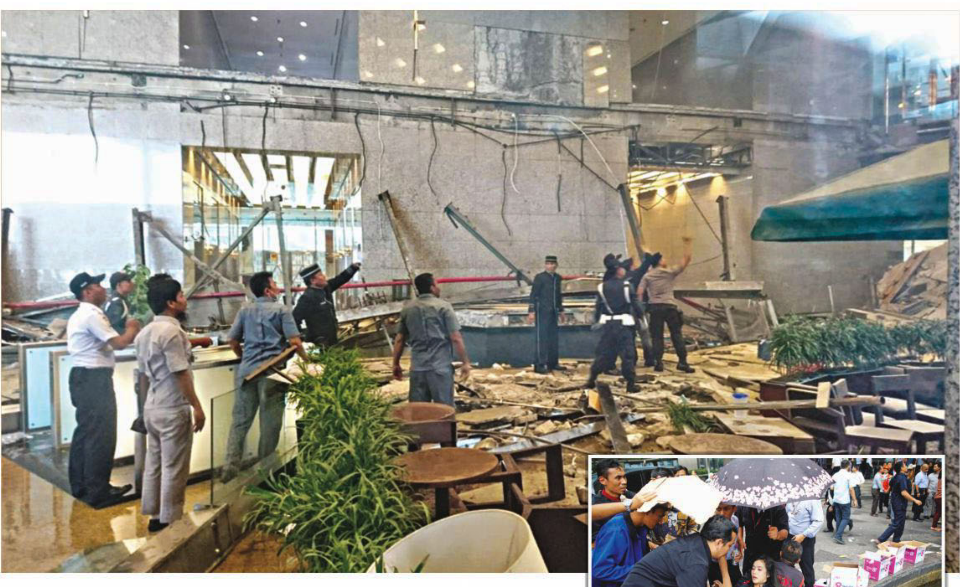
Workers and security officials examine the damage after a mezzanine floor collapsed at the Indonesia Stock Exchange building in Jakarta yesterday. Inset, people help an injured person outside the building. National police spokesman said 75 people were injured after the floor collapsed. PHOTO: REUTERS
