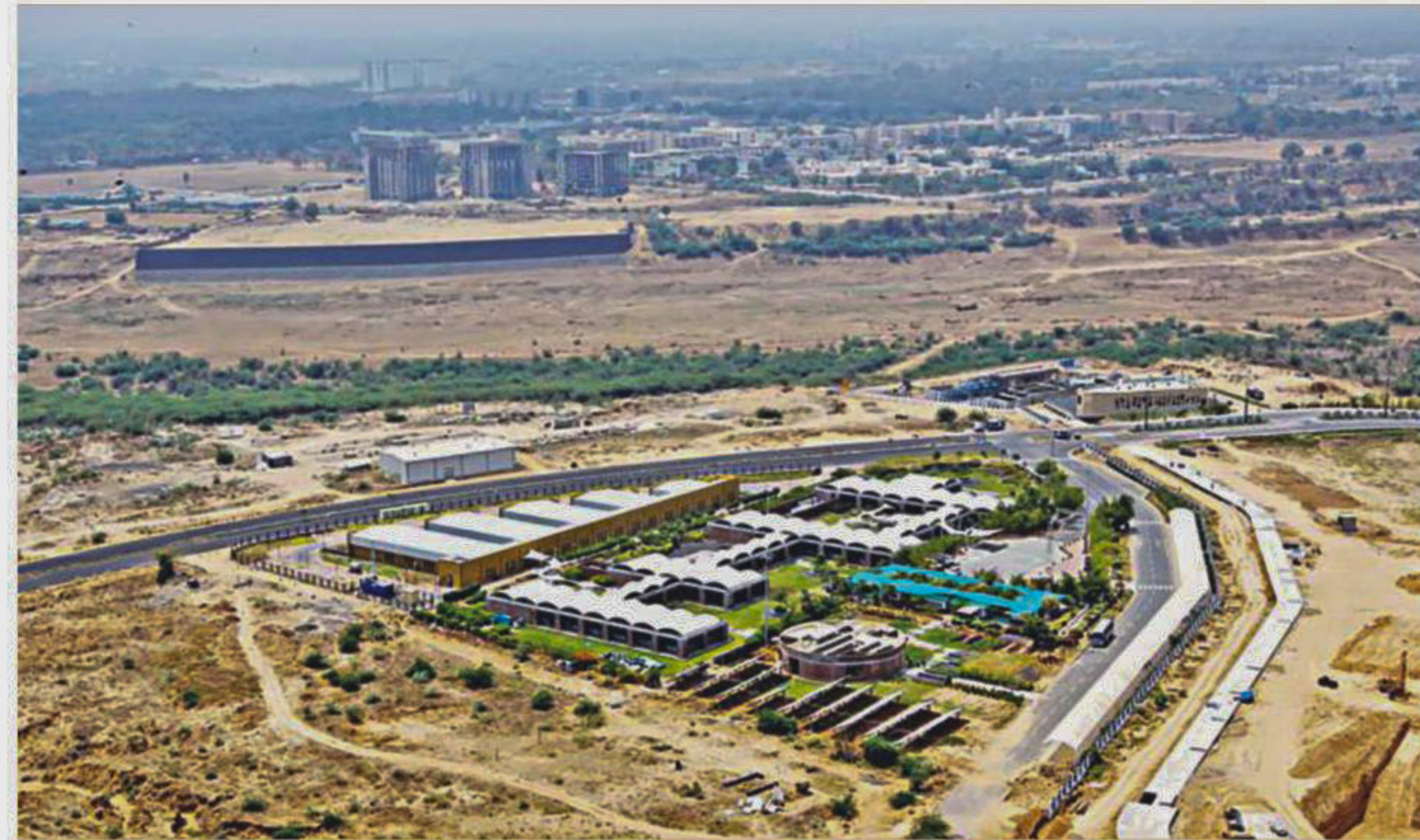
An aerial view of a site under construction at the Gujarat International Finance Tec-City at Gandhinagar in Gujarat, India. It is part of a grand scheme to build "smart" cities that the country hopes will provide a model for its urban future.
