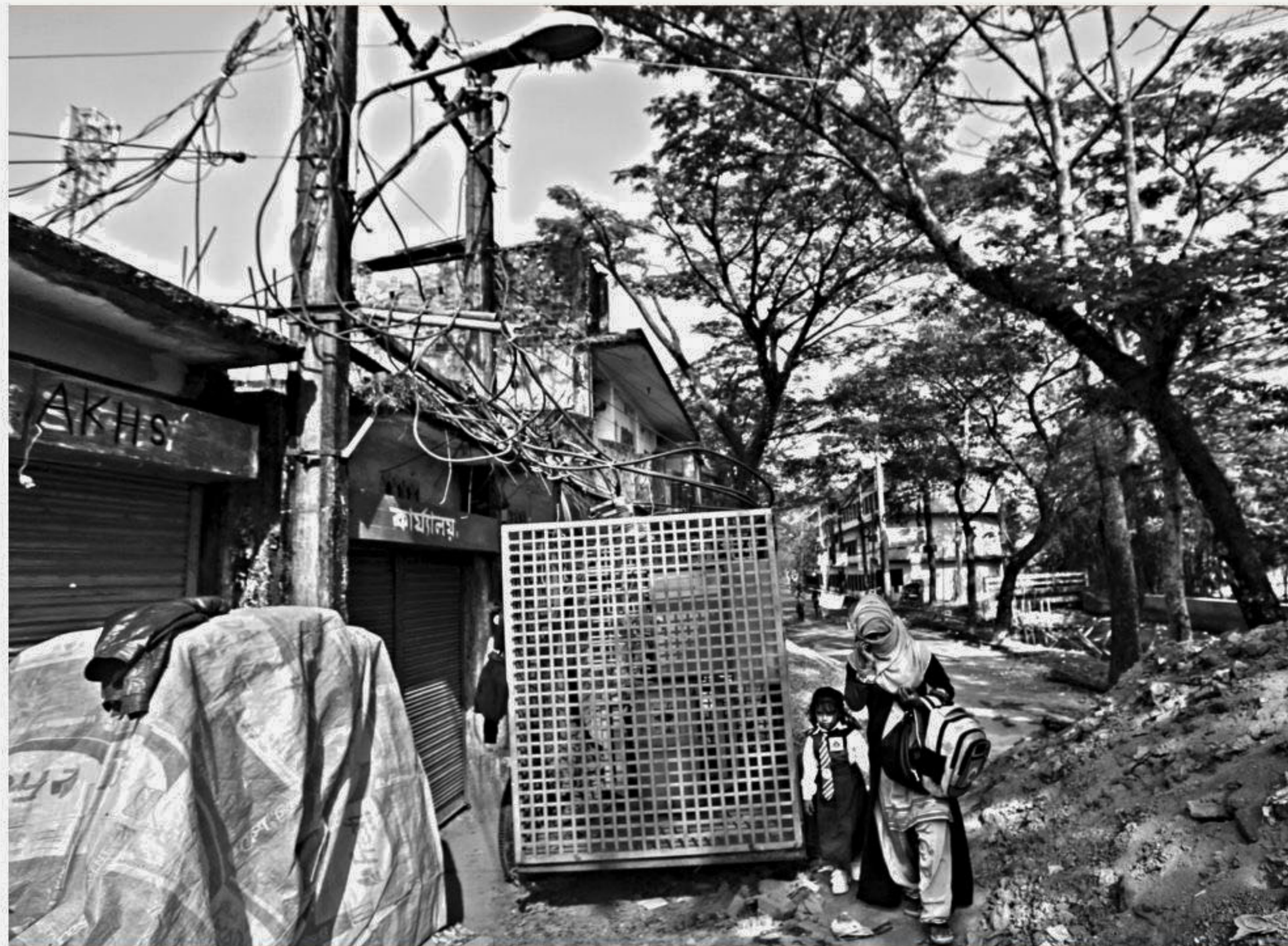
A woman and a child pass through a narrow passage available on a road where a portable transformer is parked dangerously within the reach of pedestrians. They could not avoid getting close to the transformer as a pile of earth is blocking the rest of the road. The photo was taken yesterday from Kaytorail Barokhali area of Sylhet city.
