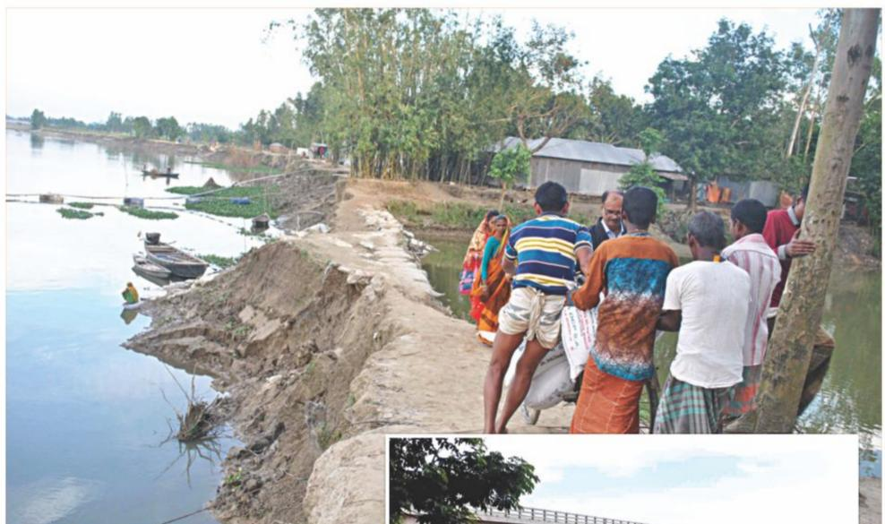
The approach road to the Trimohoni bridge on Bonarpara-Gobindaganj road is being eroded by the Karatoa river, hampering movement of vehicles. Inset, the newly-built 360-metre Trimohoni bridge over the Karatoa river.
