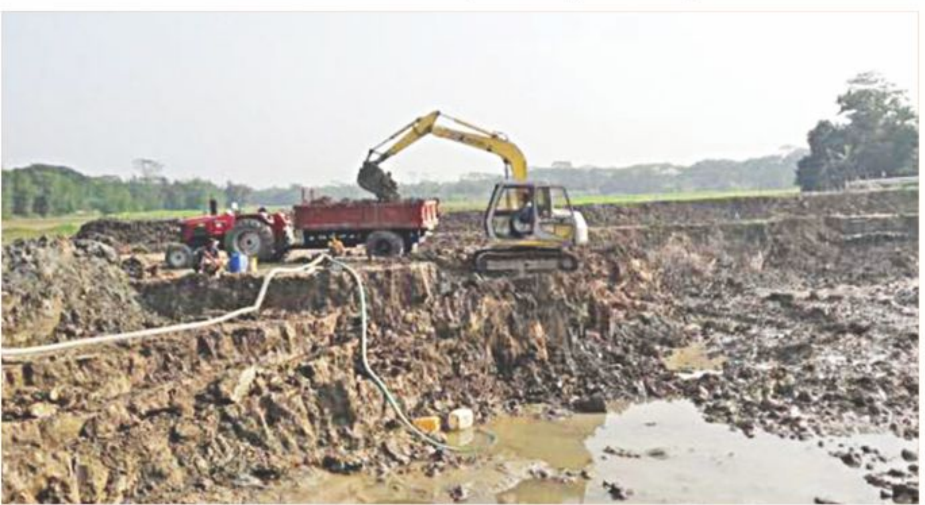
An excavator loading a tractor trailer with earth in Chandulia area of Mirzapur.
