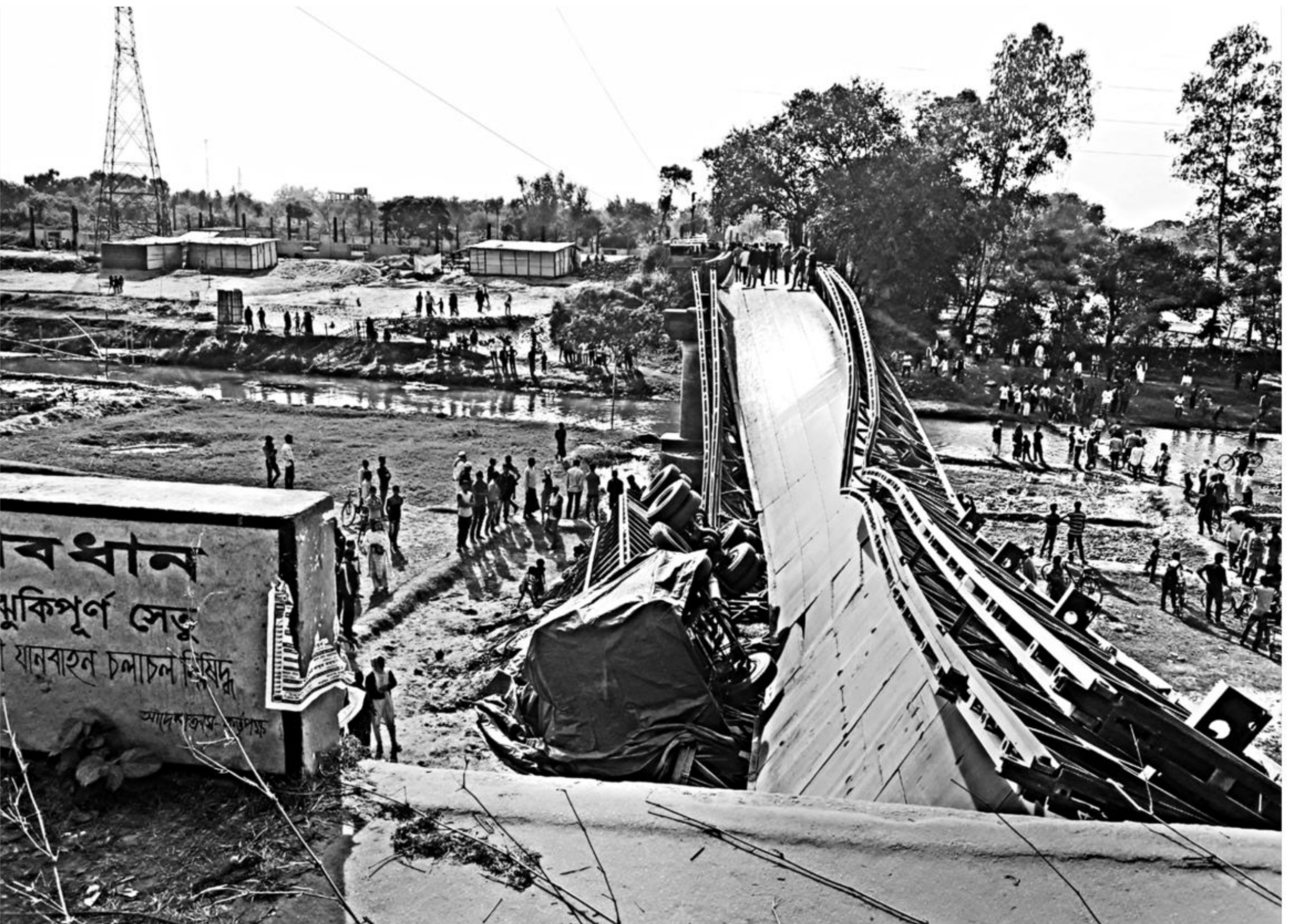
A Bailey bridge over the Senua river on Thakurgaon-Raniganj road in Sadar upazila collapsed on Friday when an overloaded truck crossed it despite cautionary notice forbidding movement of overloaded vehicles on the bridge.
