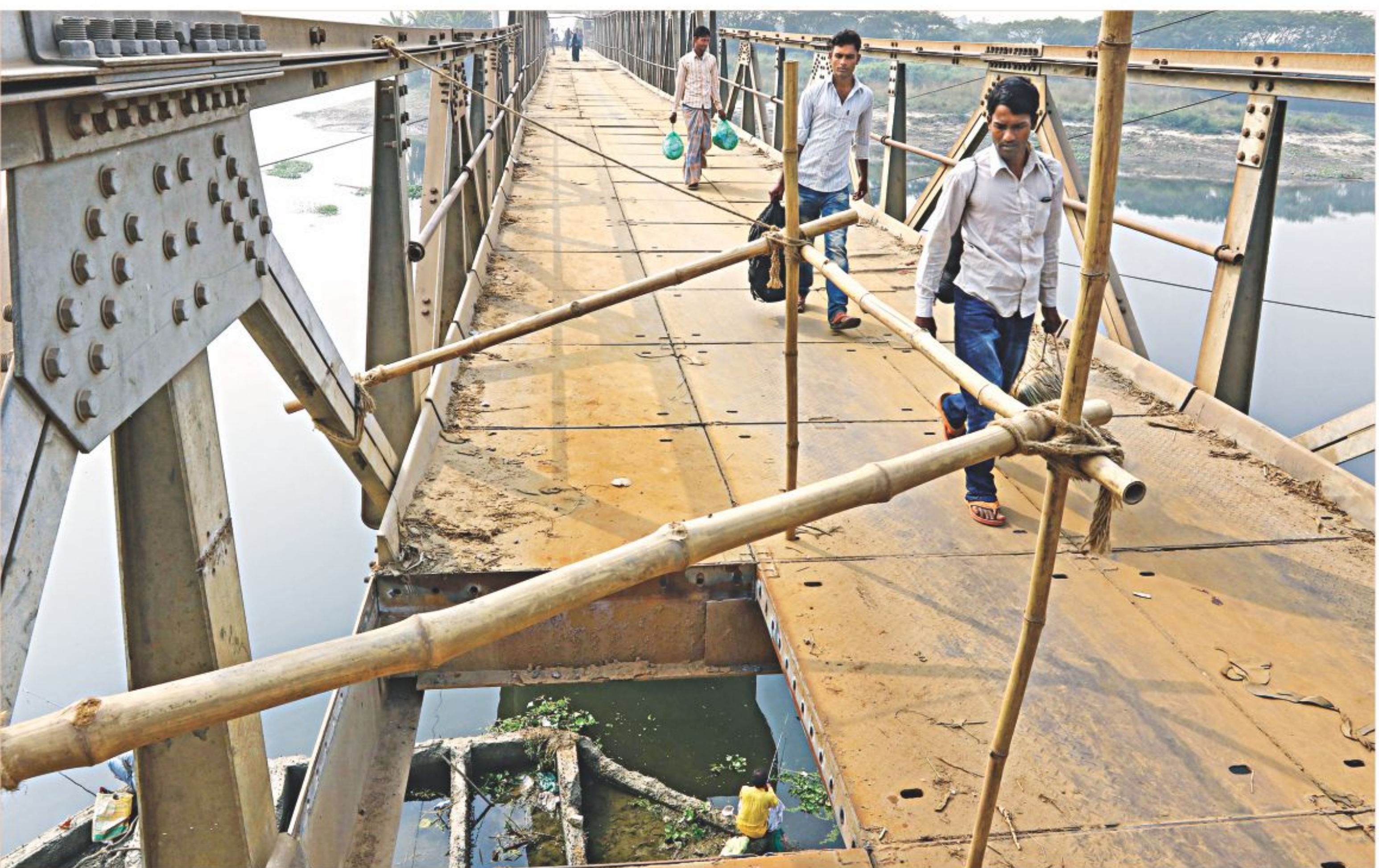
People walk on a dilapidated bridge to cross the Turag river in Savar's Bhakuta union yesterday. The bailey bridge, missing a steel section, has been lying like this for the last seven days. The rest of the metal sections of the bridge have also become rusty due to overuse. If not repaired immediately, an accident might occur any time. The photo was taken yesterday.
