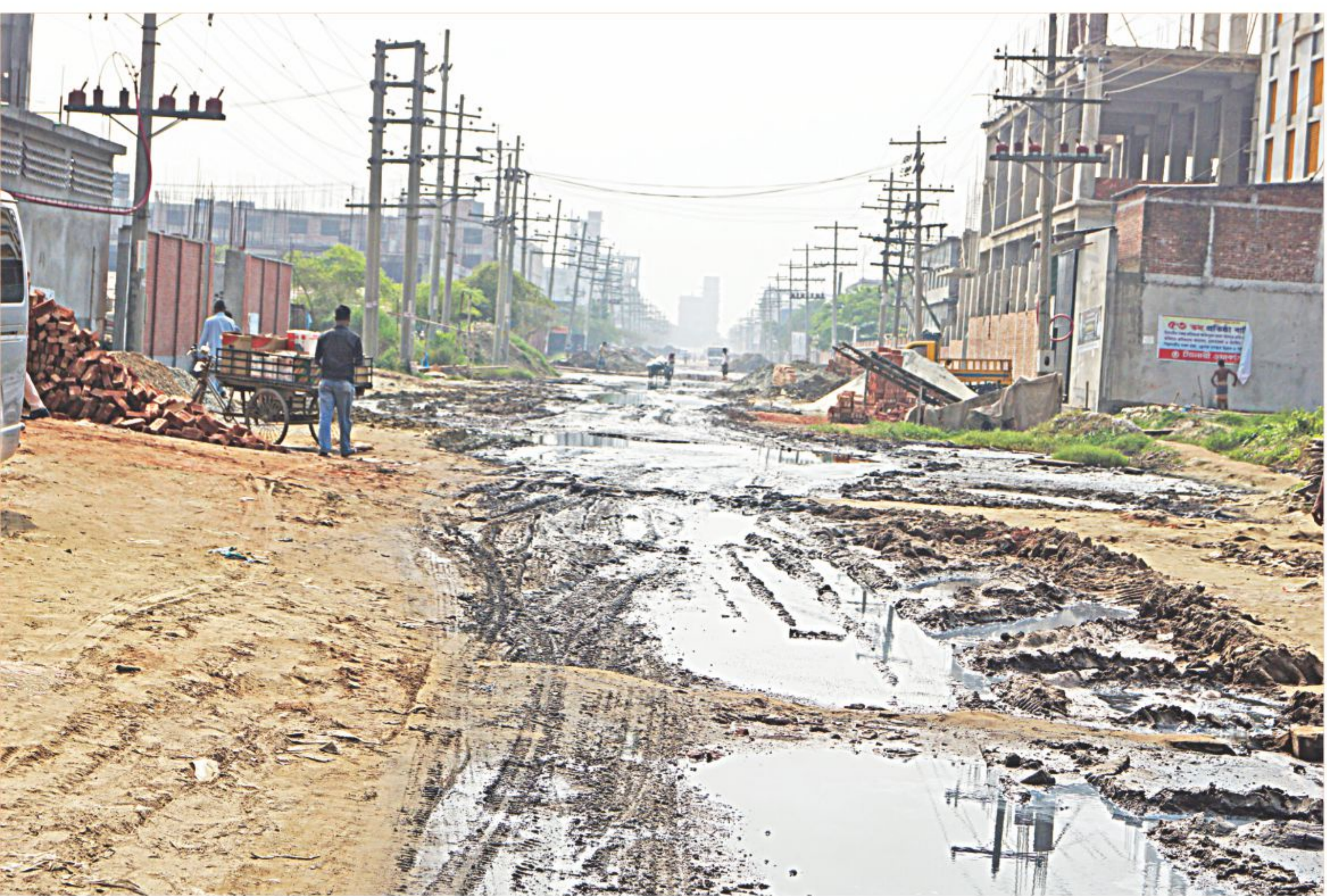
This is the main road in Savar Tannery Industrial Estate. No matter it rains or shines, the roads inside remain muddy all the time. In the absence of a proper drainage network, toxic water submerges the roads, making it difficult for the workers to move through. The photo was taken recently.
