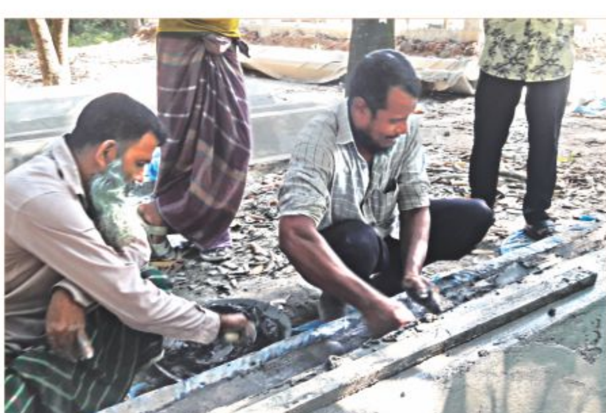
An official of the Housing and Building Research Institute demonstrates the use of compressed stabilised earth blocks at its office in the city's Darussalam area. Made of soil dredged out of rivers and cement, this alternative brick is produced without baking in kilns reducing pollution and destruction of arable land. It can cut construction cost by around 30 percent. Bottom left, a five-storey model building, built with alternative building materials, at the institute. Bottom right, workers make low cost roofing plates that can replace sheet metal roofs. The photos were taken last week.
