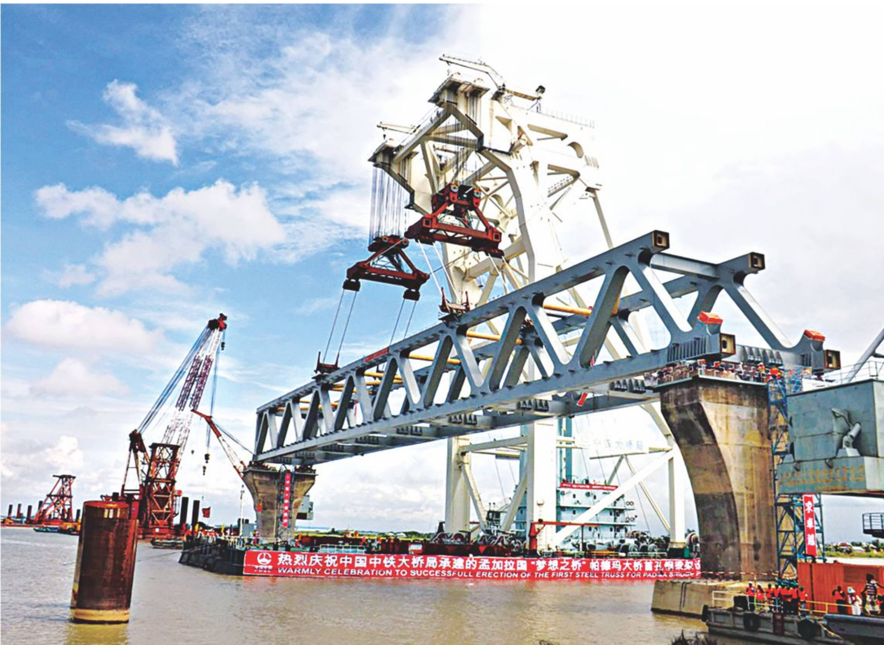
The installation of the first of 41 spans on piers of the Padma Bridge was completed yesterday. The photo was taken at Shariatpur's Zajira.
