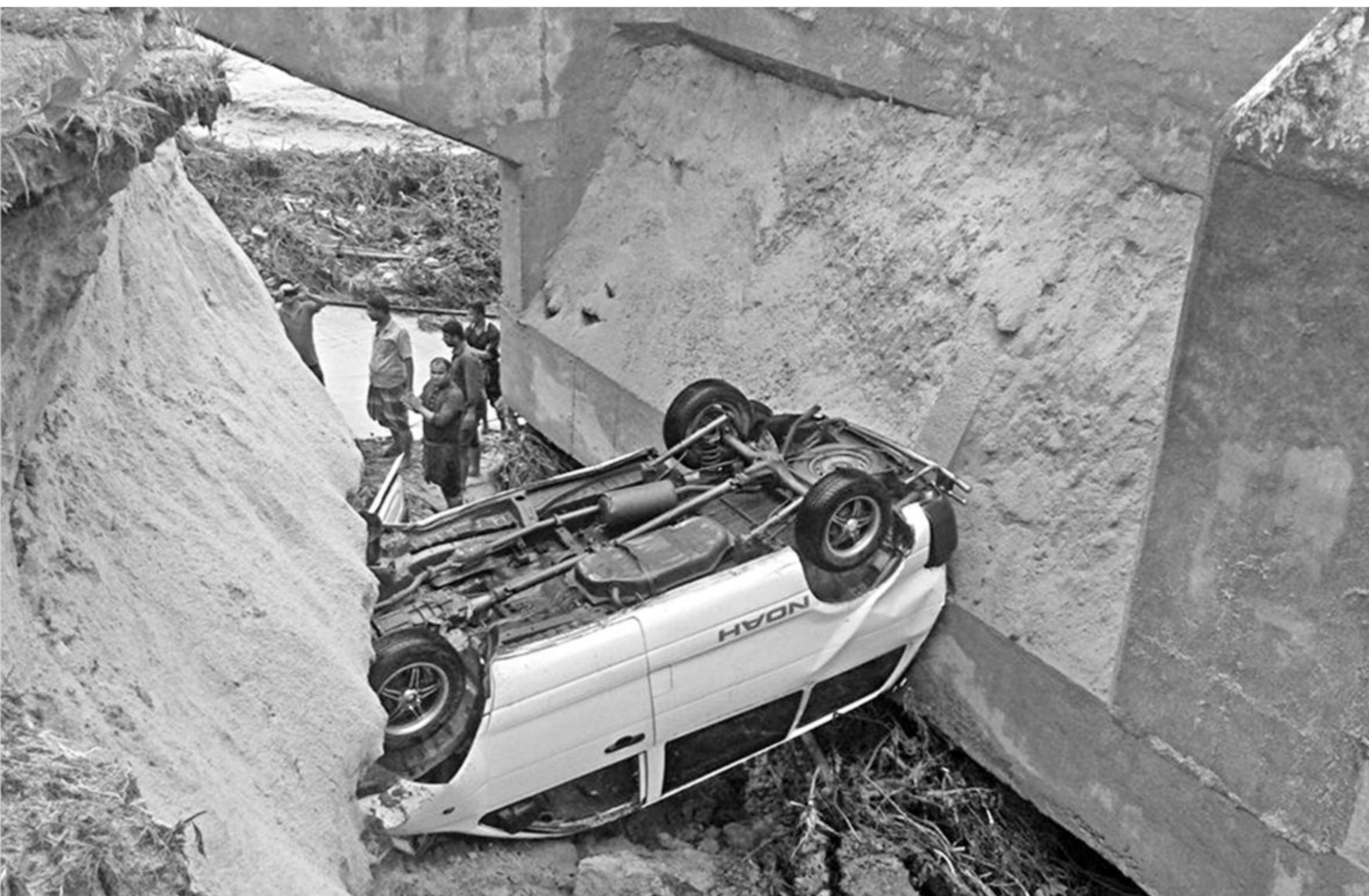
This microbus fell into the gap between the bridge and the approach road, created by illegal sand lifting and heavy rain in Chunarughat upazila of Habiganj.
