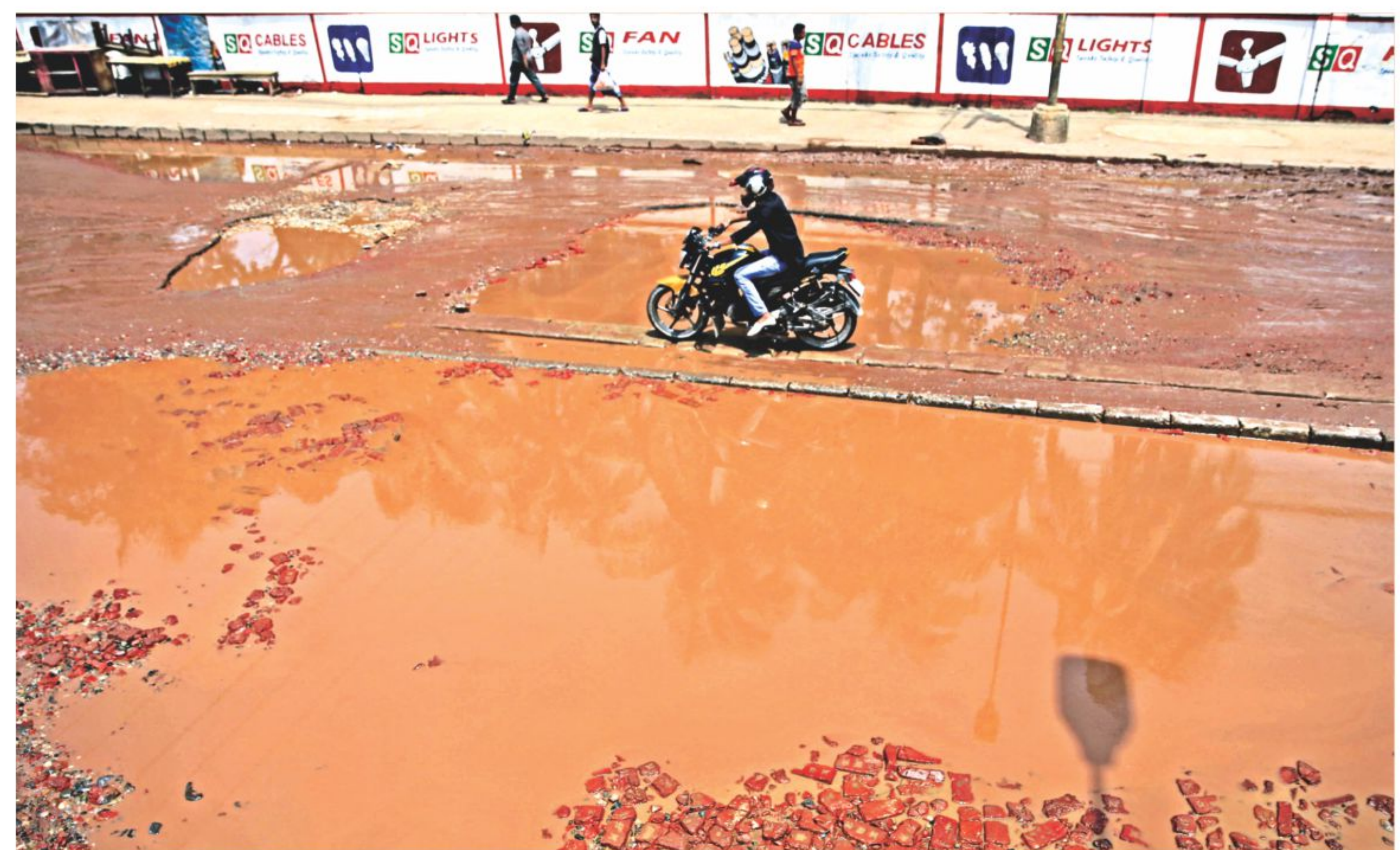
As in the case of most other roads, this road near Postogola Fire Station also became damaged during this monsoon as it lacks a proper drainage system. A large amount of money on frequent repair works could be saved if the authorities ensured a functioning drainage for every road. The photo was taken yesterday.
