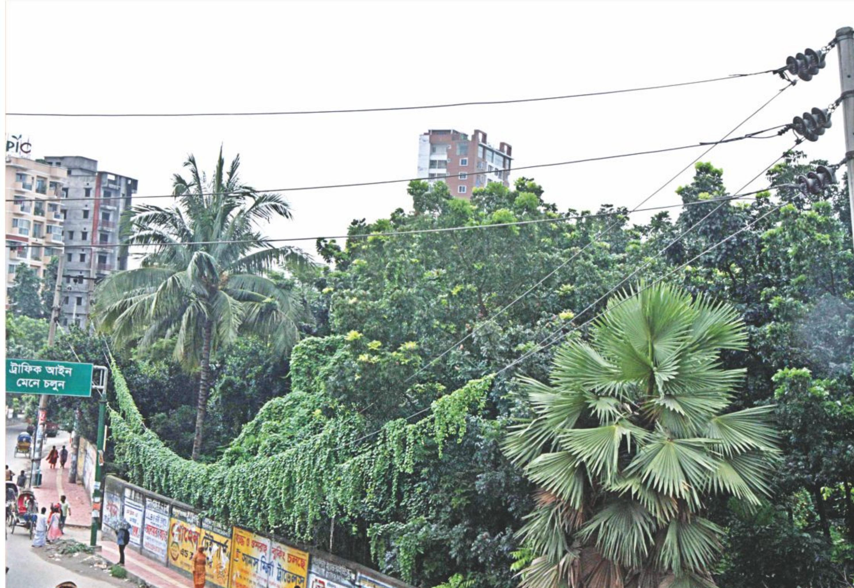
Shrubs cover high-voltage power cables in Bashabo near Khilgaon Flyover and bring them close to the pavement. The weight has caused the electric poles to lean to one side. This may cause an accident any time.
