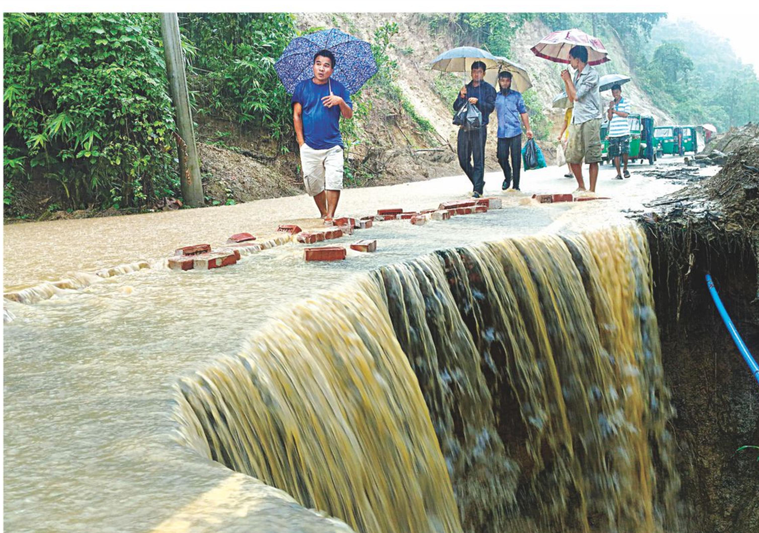
This part of the Rangamati-Khagrachhari Link Road was washed away by heavy rains in Sapchhari area of Rangamati in the early hours yesterday, stopping vehicle movement. This road was also badly damaged during the landslides in the district on June 13, but the Roads and Highways Department repaired and opened it to light vehicles recently.
