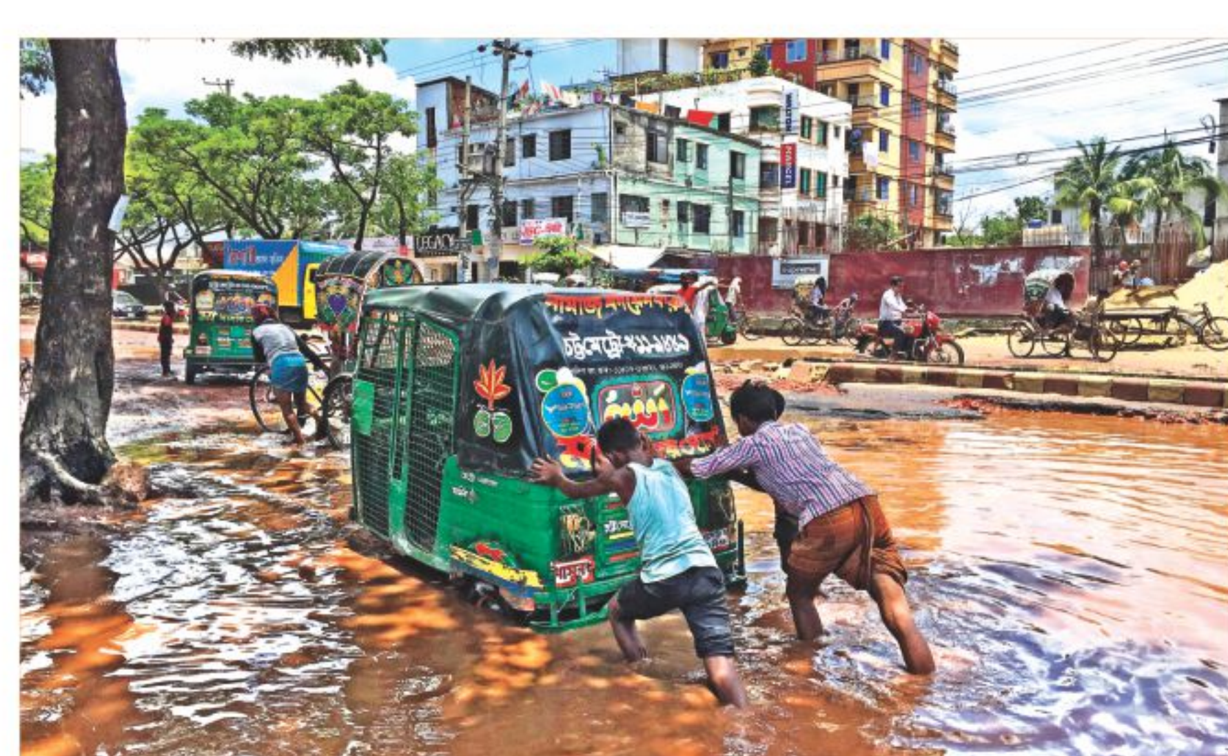
This is Agrabad Access Road -- a major thoroughfare in Chittagong city. The road developed large potholes as it remains under tidal water almost all year round. The situation took a turn for the worse with torrential monsoon rain. The potholes gradually became larger and took shapes of craters. Many vehicles malfunction while trying to cross this portion of the waterlogged road every day. The photos were taken yesterday morning. PHOTO: ANURUP KANTI DAS
