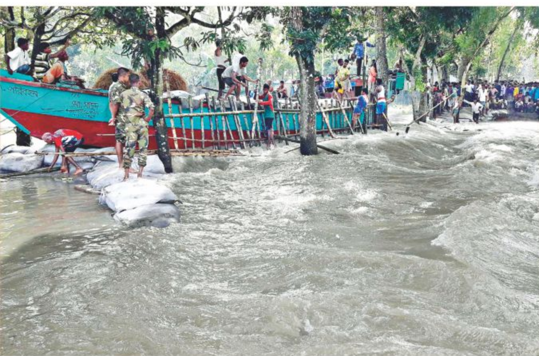
A joint team of army and the Water Development Board repair a flood control embankment at Bahuka in Sirajganj after a part of it was breached by the onrush of waters of the Jamuna River Thursday night. The river has been flowing above danger level flooding areas of the northern region of Bangladesh. The photo was taken around noon yesterday.
