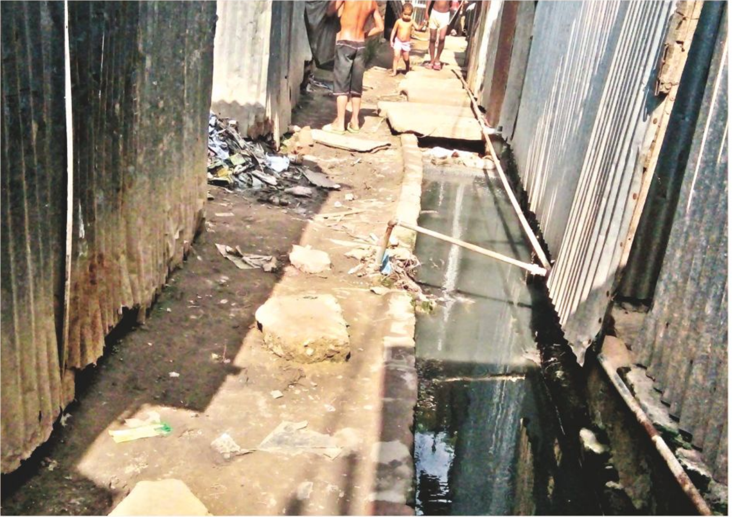
This pipe, which at first appears to be a water line, is actually used for supplying gas. The rust makes it vulnerable to leaks which can result in tragedy. The photo was taken recently.
