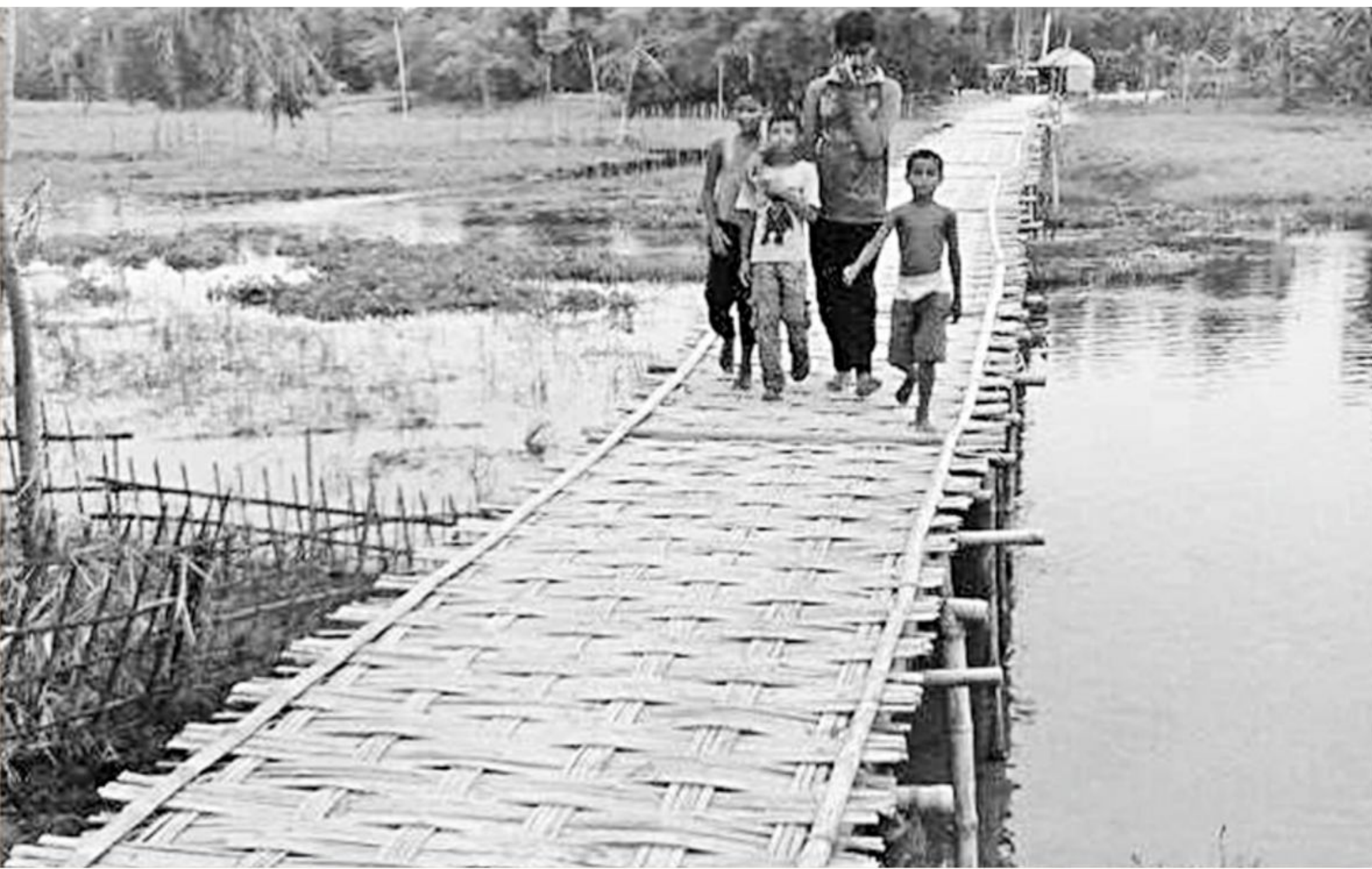
Villagers have built a 400-foot-long bamboo bridge over the Sati river in Kaunia upazila of Rangpur to ease sufferings of residents of seven villages.
