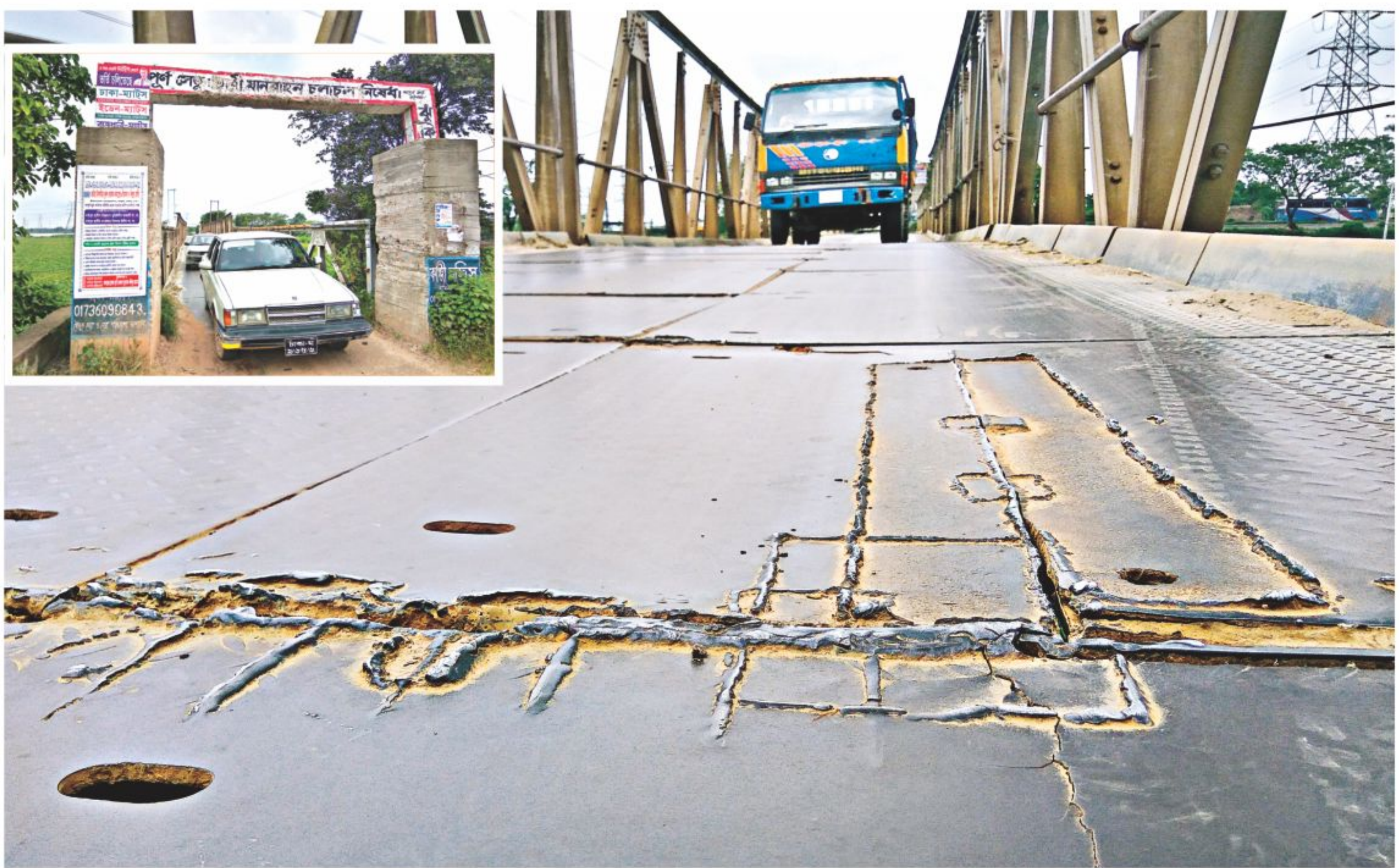
A car crosses the rickety Bhakurta Steel Bridge over the Turag river in Savar. A large sign on the bridge, inset, forbids heavy vehicles from using it. The 379-foot bridge has been in a dilapidated condition for years. But heavy vehicles still use the risky bridge as the authorities concerned have apparently done nothing yet to repair or rebuild it. The Daily Star published similar photos of the bridge before, mentioning the risks involved. The photos were taken on Wednesday.
