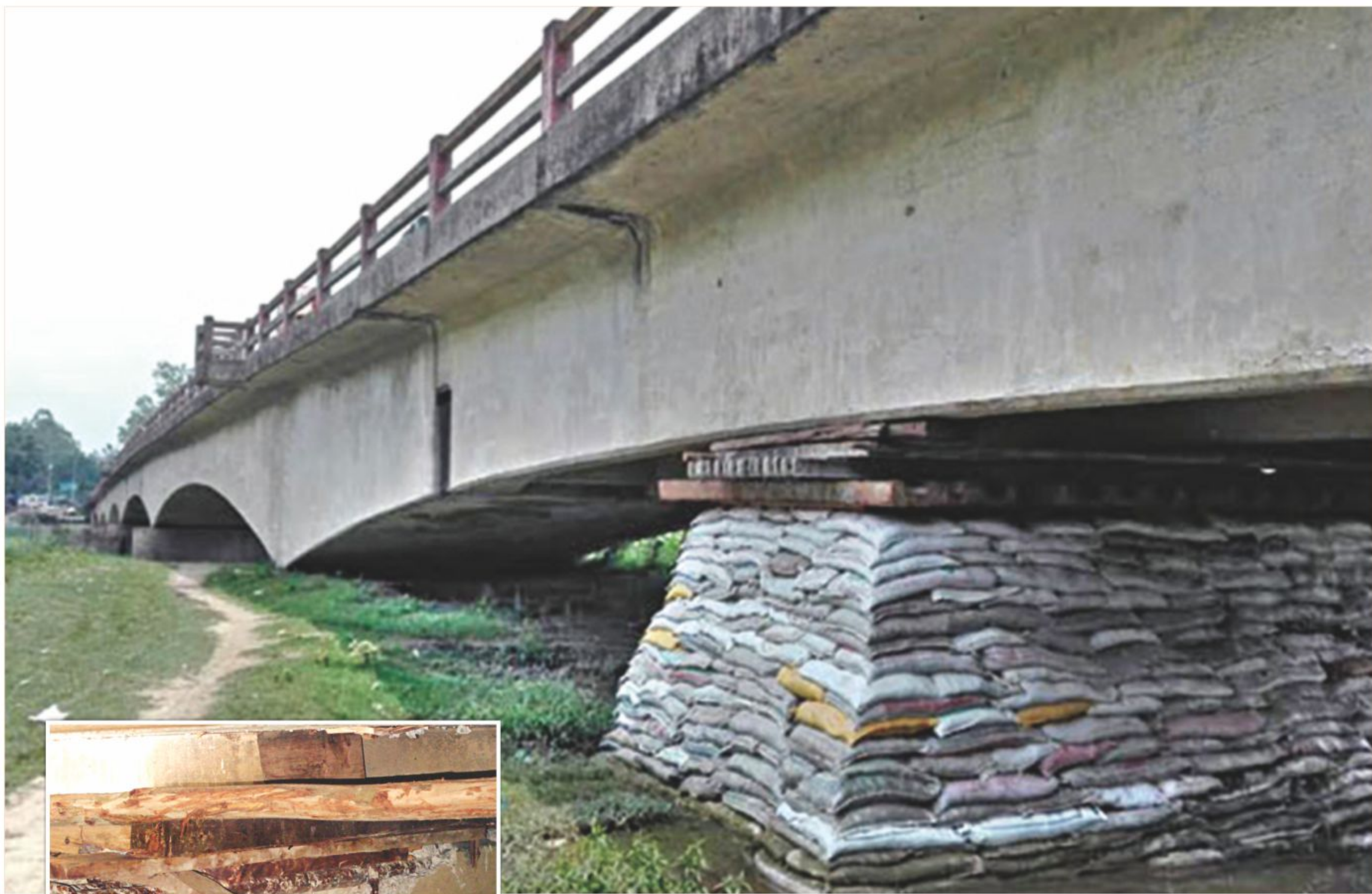
With the middle portion precariously sagged, Matamuhuri Bridge on Cox's Bazar-Chittagong road in Chakoria upazila under Cox's Bazar district lies in an awful state for the last couple of years, putting vehicles plying the nationally important road vulnerable to serious accident anytime. Inset, awkwardly set timber at the broken portion of the bridge deck.
