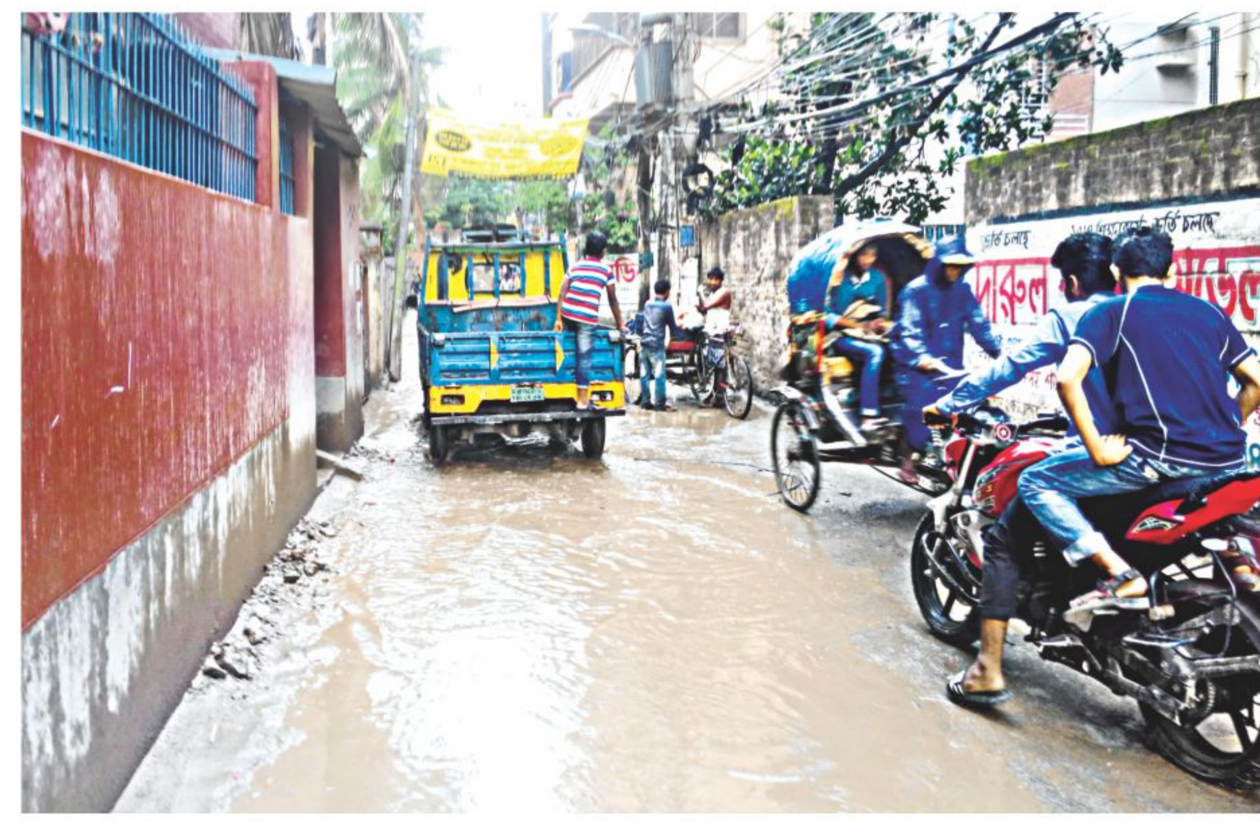
THE ROAD FORGOTTEN... This unmaintained road, Tally Office Road near Wasa old pump in Rayer Bazar, is used by thousands who live in the low-priced housings on both sides of Beribadh (embankment) road near the martyred intellectual memorial. The decaying of the road started about 15 years ago when the authorities replaced its perfectly-working open drain with a narrow underground pipeline. Over time, indiscriminate dumping of garbage clogged up the pipeline. Now, with no drainage system in existence, the road is dotted with hundreds of small to medium potholes where ankle-deep puddles of water are created even after a light shower. During the dry season, the road is blanketed with a cloud of dust -- a source of respiratory diseases common in almost every household in the area. The photo was taken on Wednesday. PHOTO: FIROZ A MUZHAFID
