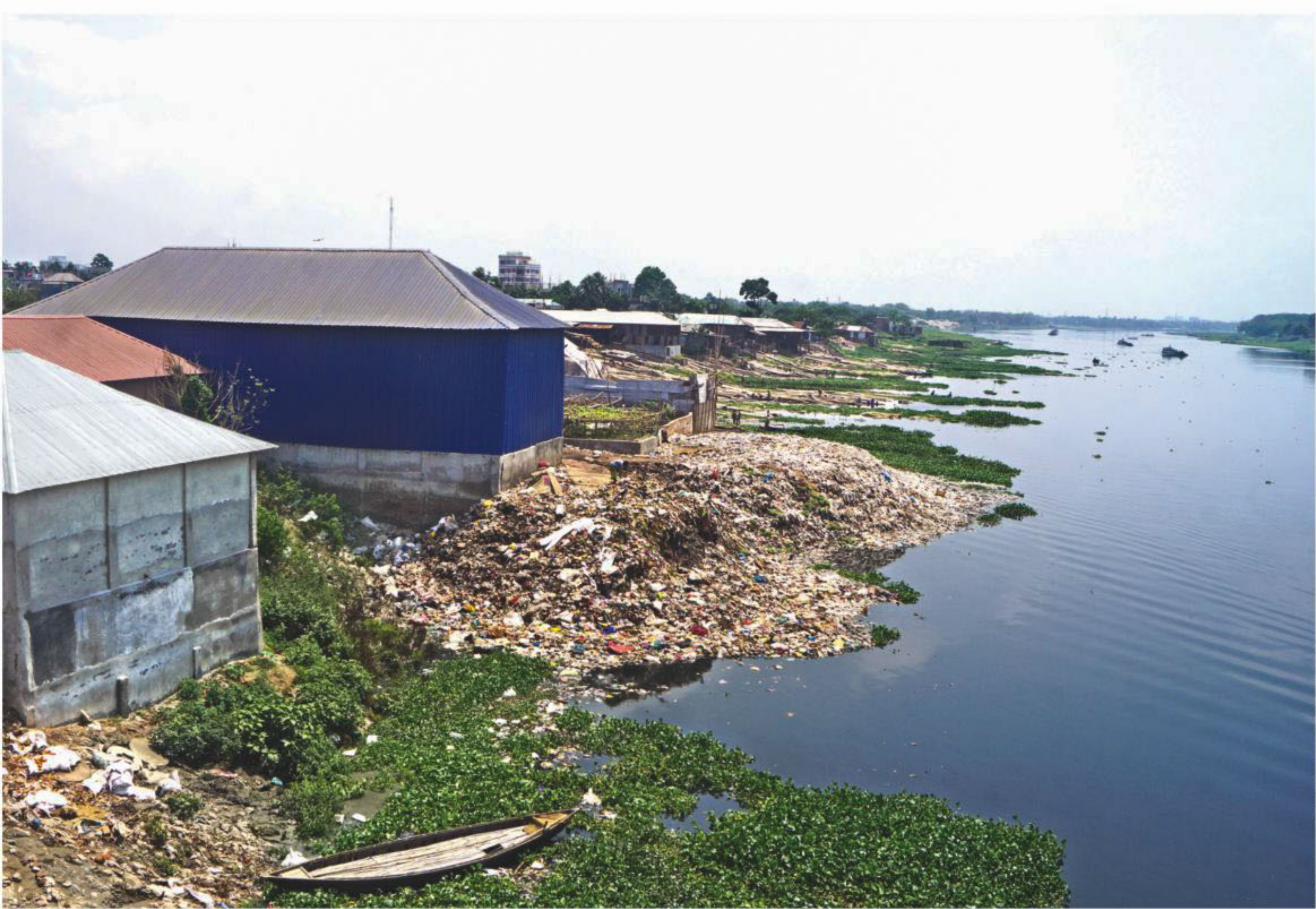
Business establishments set up encroaching upon the Bongshi river in Namabazaar area of Savar. The grabbers have been in the business for years whereas the authorities concerned continue to turn a blind eye to the illegal practice. Apart from the mindless encroachment, different industrial units are also dumping effluents into the river, rendering a blow to the aquatic life. The photo was taken recently.
