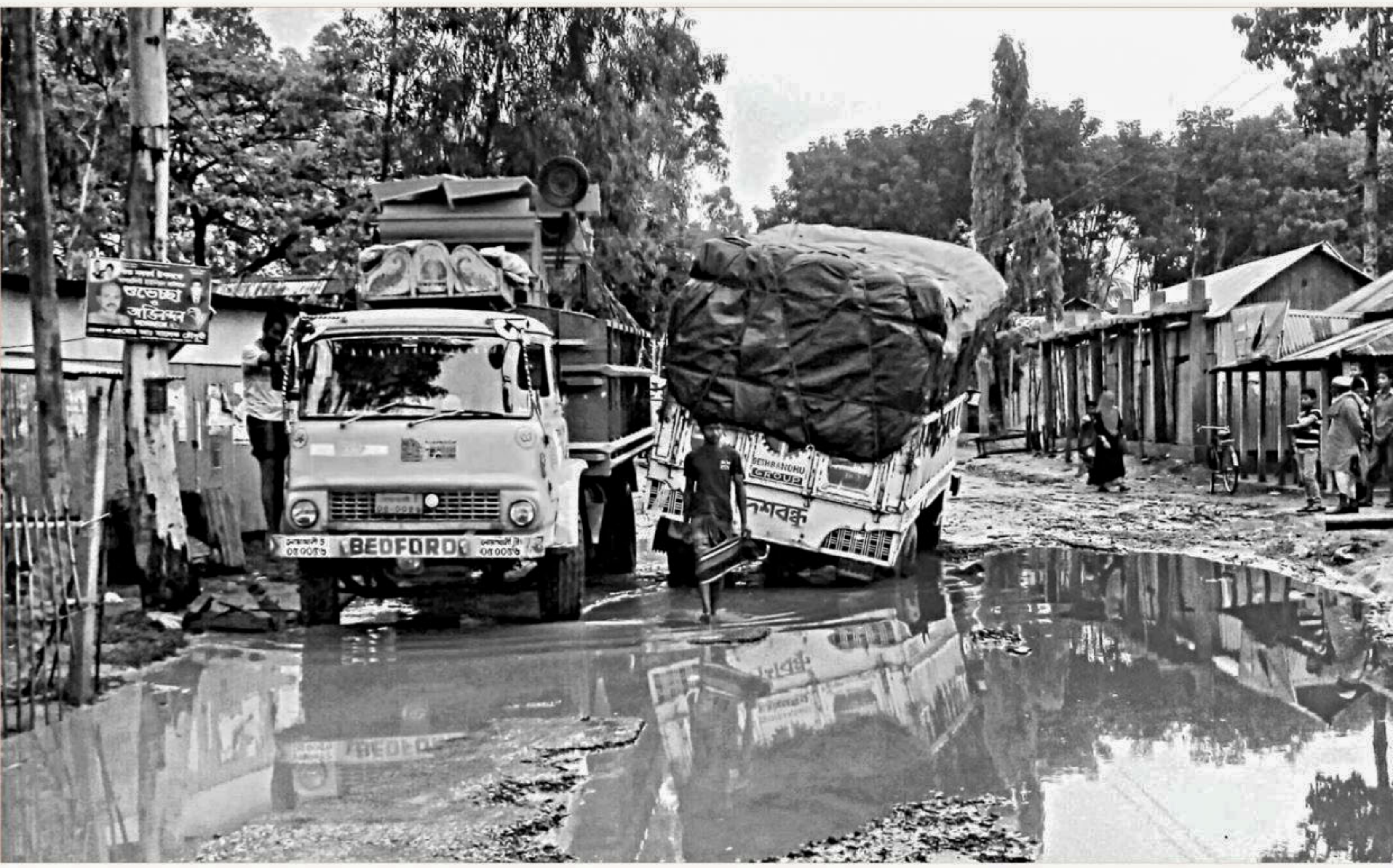
Two trucks get stuck in a huge pothole on Ghtail-Guptabrindabon road in Tangail. The 30km road is in extremely bad shape and in need of repairing. At night, passengers and transport workers often become victims of mugging when their vehicles get stuck in potholes.
