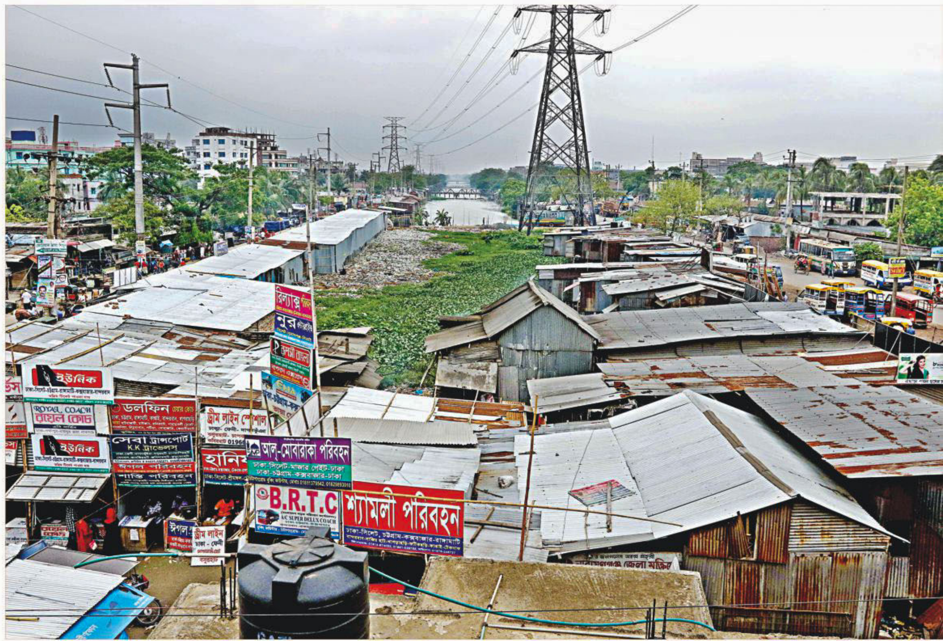
The DND canal adjoining Dhaka-Chittagong highway in Narayanganj's Shimrail is being choked to death, as a group of unscrupulous traders continue to build illegal structures, encroaching on the water body. There is hardly any initiative by the authorities to free the canal from the clutches of the grabbers.
