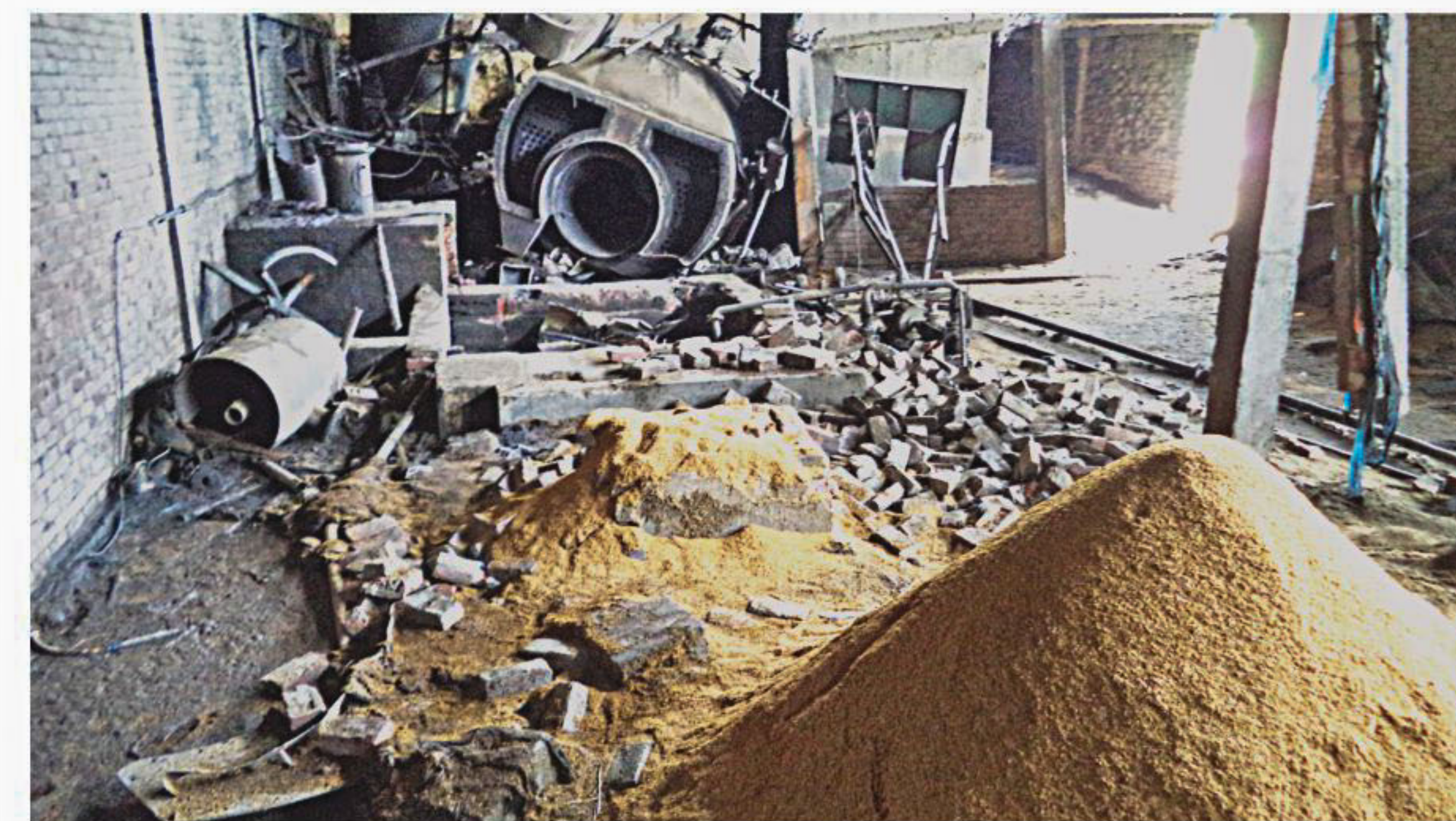
Machineries lay damaged at Jamuna Automatic Rice Mill in Dinajpur's Gopalganj area. A boiler explosion at the mill on April 19 left 13 people, including a woman, killed. Fourteen injured workers were undergoing treatment at M Abdur Rahim Medical College Hospital (previously Dinajpur Medical College Hospital) and Rangpur Medical College Hospital.
