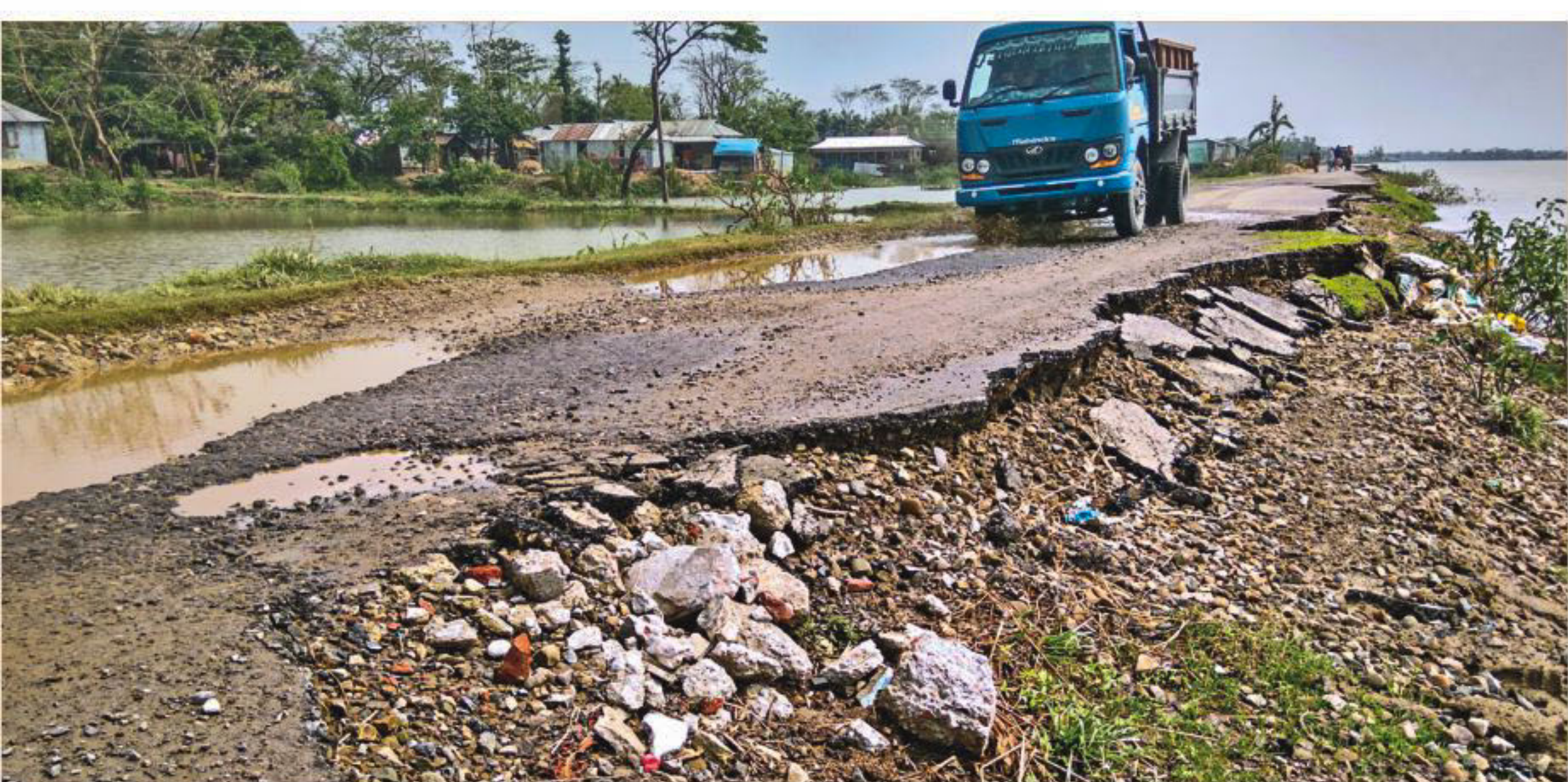
A truck goes over a puddle on the rundown Airport Bypass Road built on an embankment alongside Chamaurakandi Haor under Sadar upazila of Sylhet. Flash floods caused by last month's incessant rain and onrush of water from upstream rivers destroyed almost all embankments and the roads built on those in Sylhet and three other neighbouring districts. The photo was taken on Thursday.
