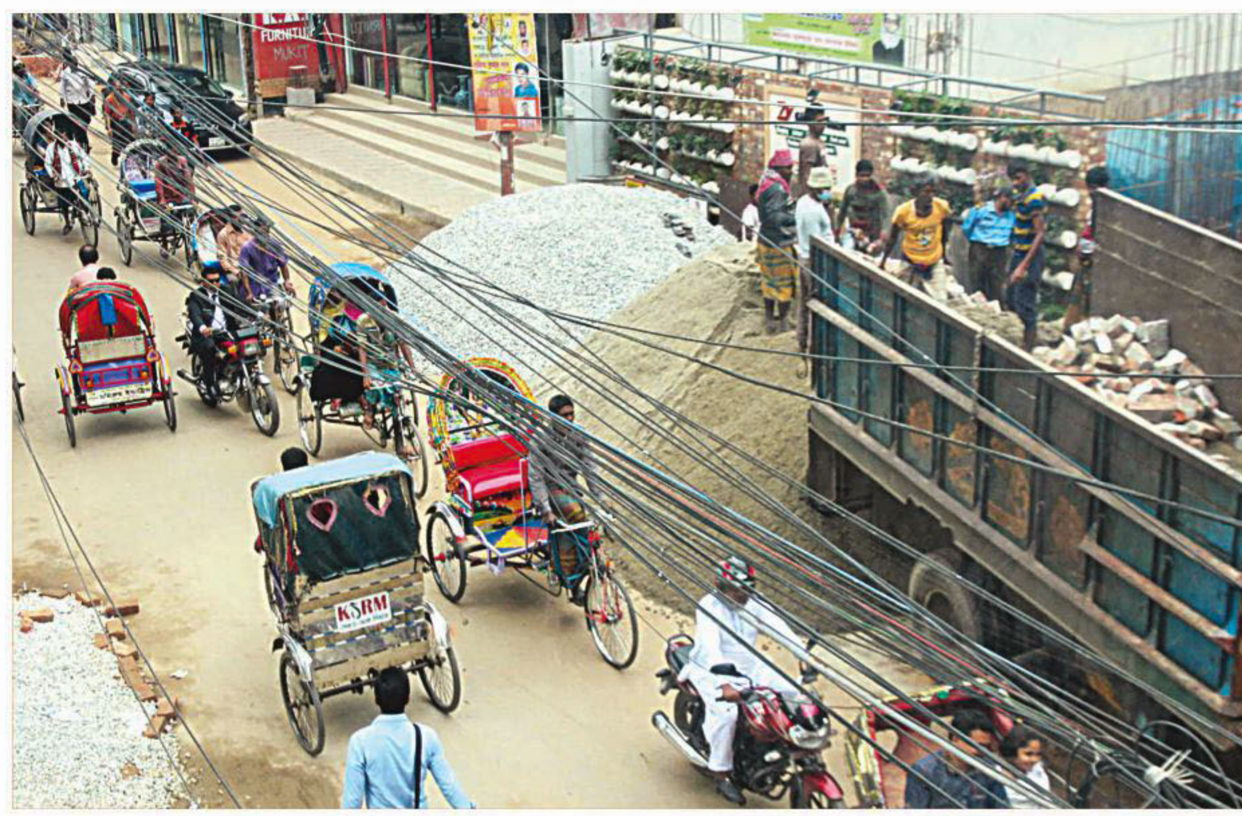
Construction materials occupy a large portion of Shaheed Abdul Jabbar Road (popularly known as VIP road) in Bogra town, causing nuisance for commuters and pedestrians on the important thoroughfare.
