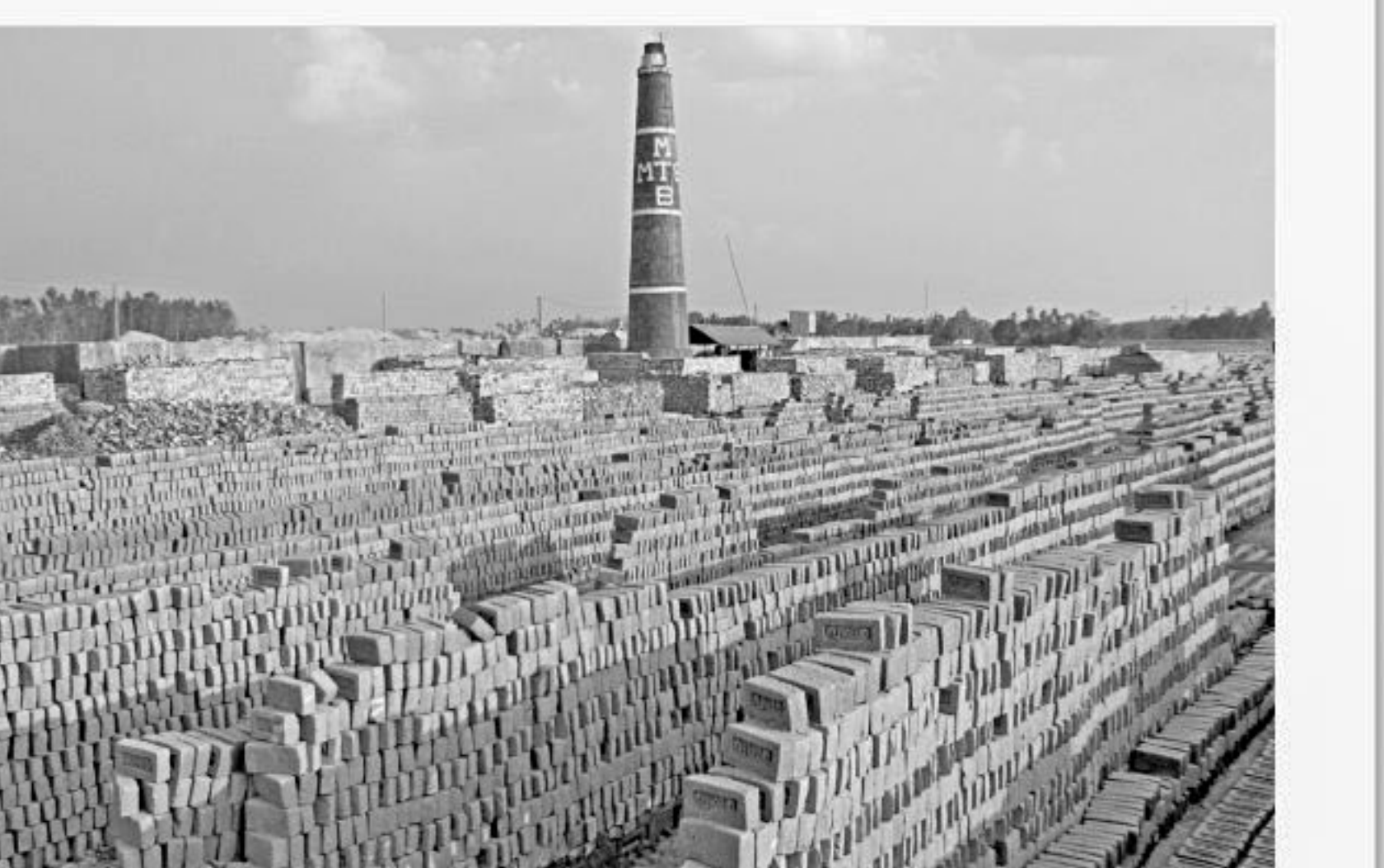
A section of unscrupulous brick kiln owners in Lalmonirhat are cheating the customers by manufacturing and supplying bricks that are smaller than the standard size, defying the government manual.
