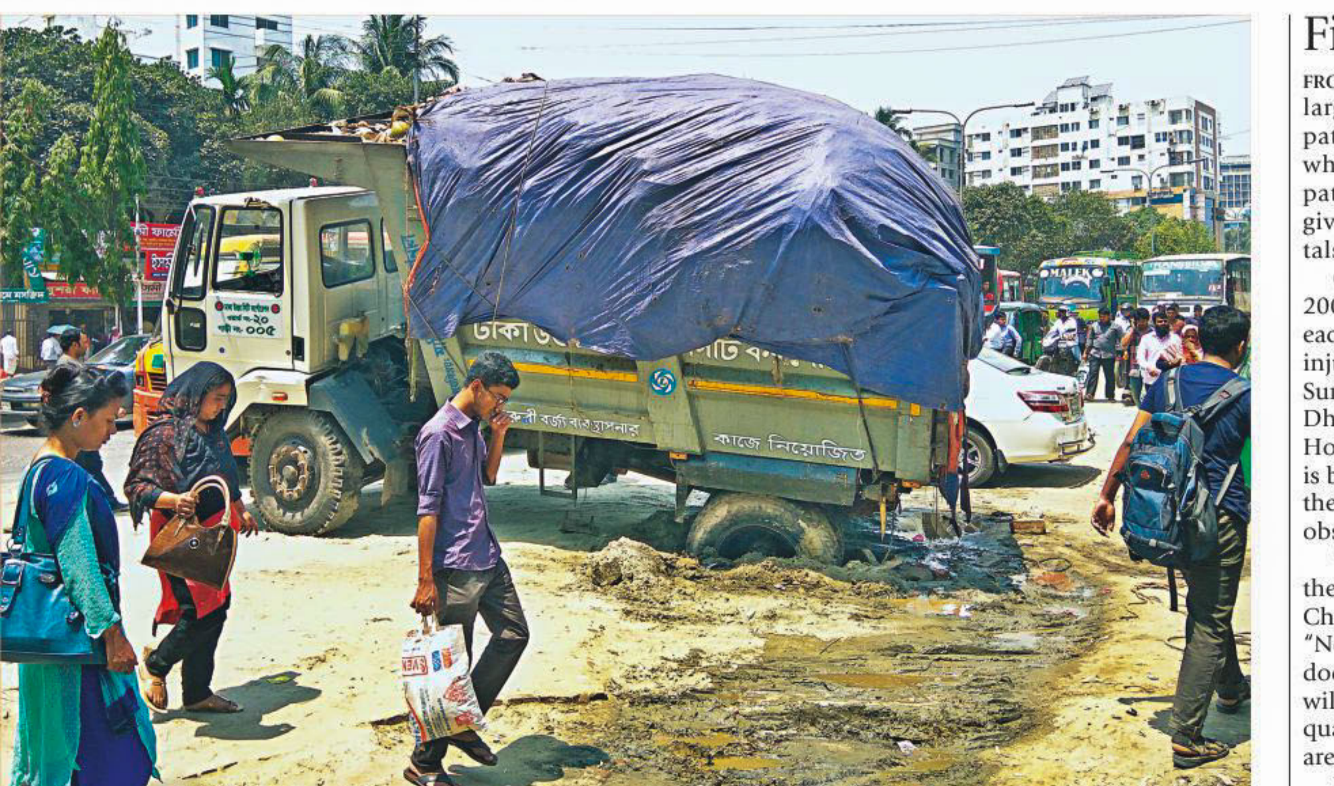
A garbage truck belonging to Dhaka North City Corporation gets stuck in sand used for filling up a portion of the capital's Mirpur Road near Suhrawardy hospital. The road was previously dug to repair the area's drainage system. Eventually the vehicle was able to get out with assistance. The authorities concerned apparently did not follow proper procedures to fill up the space, which might lead to more serious accidents. The photo was taken yesterday afternoon.
