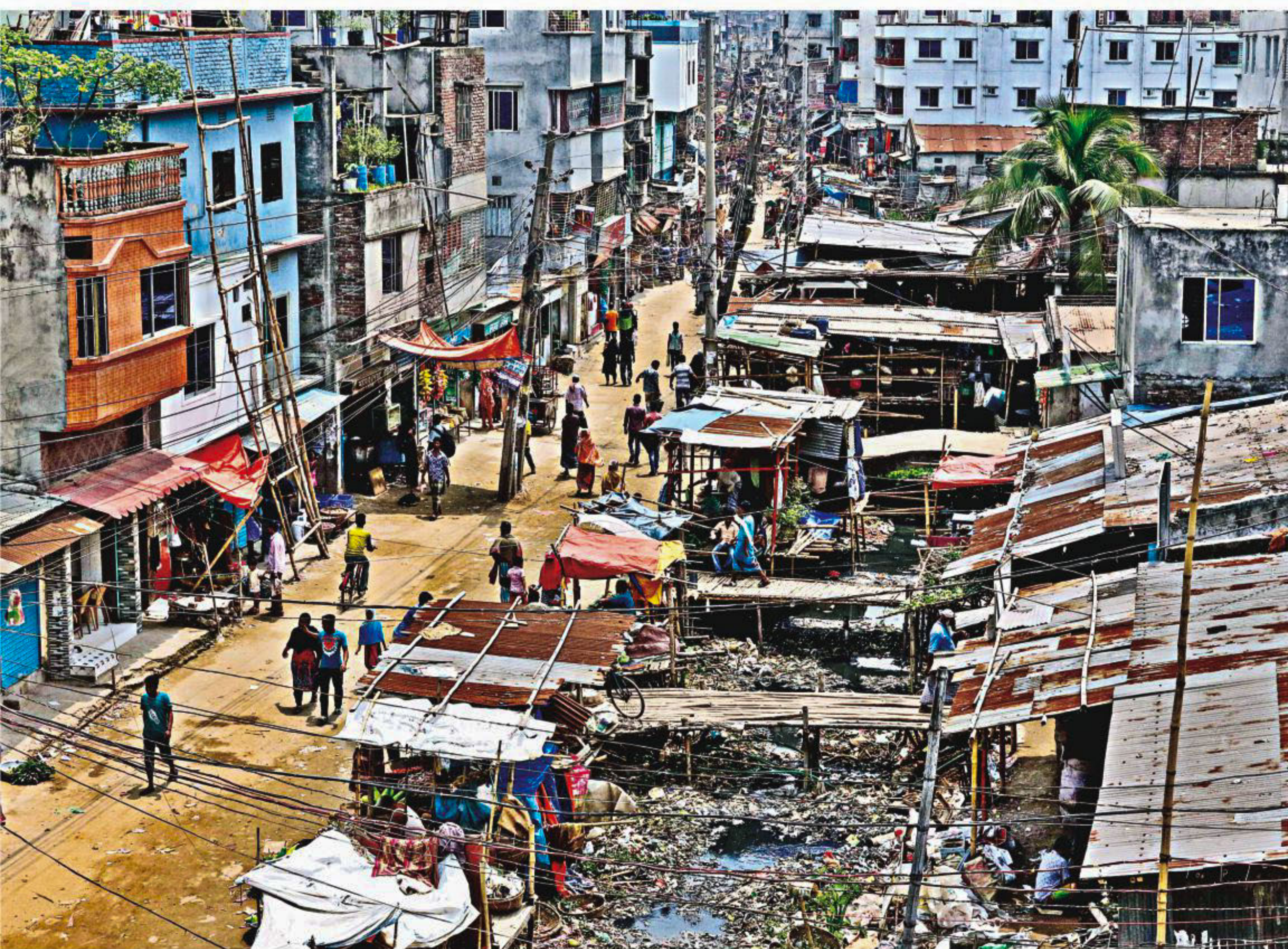
The canal, in the photo taken recently, at Deb Dholaiakhal in Dhaka is being clogged up with waste thrown by locals. Some local influential people have also filled it up partially to set up structures.
