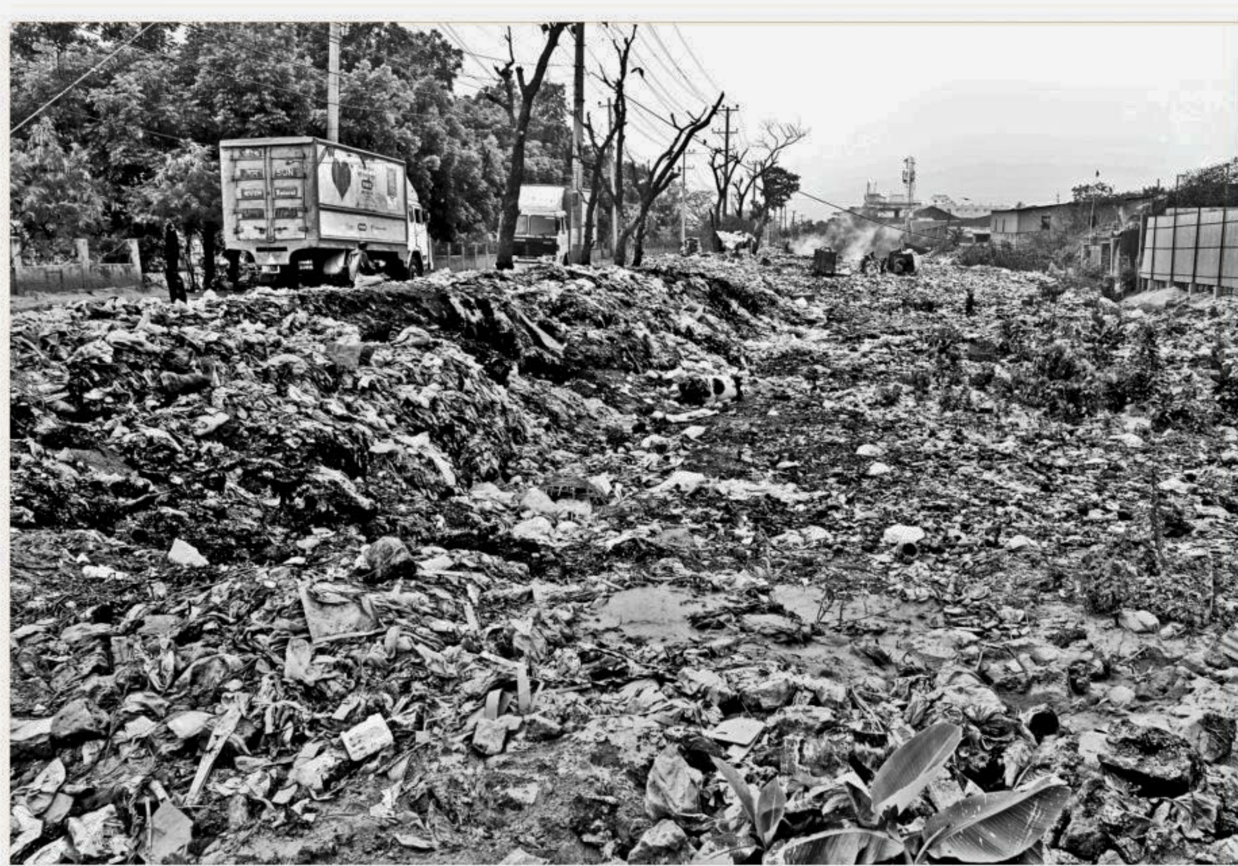
Garbage totally blocks the DND (Dhaka-Narayanganj-Demra) canal in Deilya area of the capital, while influential locals keep pressing ahead with grabbing its banks. The 4.5km canal was built in 1964 for flood control, irrigation, and drainage, but all these purposes have been frustrated. The cost of this canal being lost will be flooding in surrounding areas including in Dhaka city. The photo was taken last week. PHOTO: ANISUR RAHMAN
