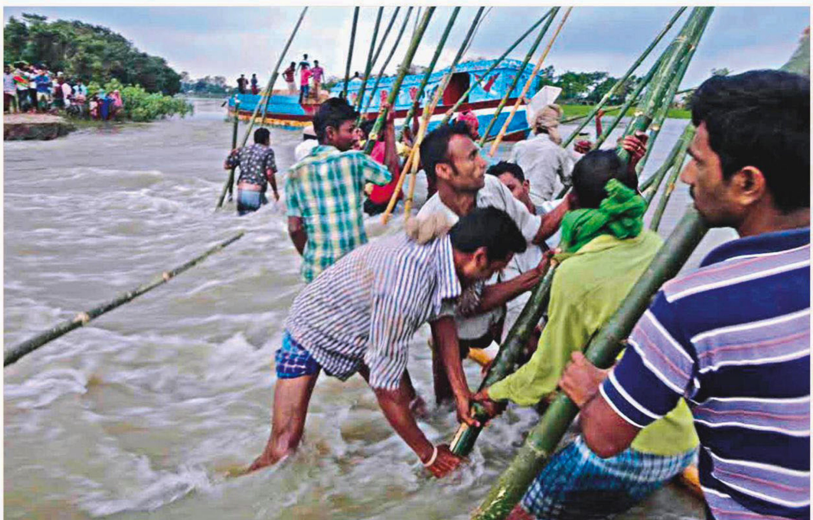
Fighting the onrush of flash flood, locals use bamboos trying to erect a fence for sandbags to save an embankment in Khorsar Haor in Sunamganj's Bishwamvapur on Thursday. However, it was of little use. Most of the Boro fields in the district went under water after heavy rain and the onrush of water from the hills breached embankments causing loss of crops.
