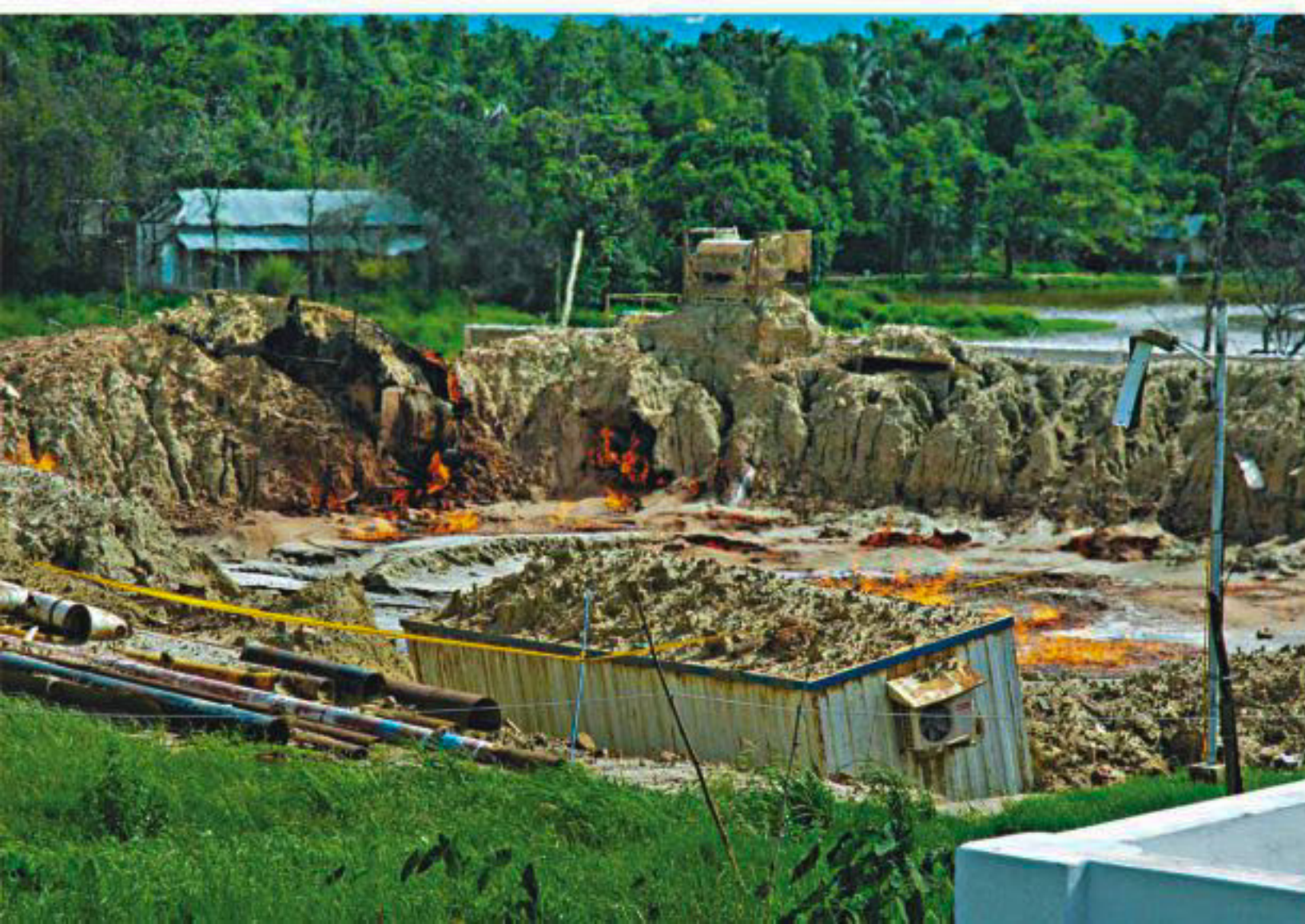
The photos taken in 2005 show gas bubbles at a waterbody near Tengratila gas field in Sunamganj and leaking gas catches fire inside the gas field.
