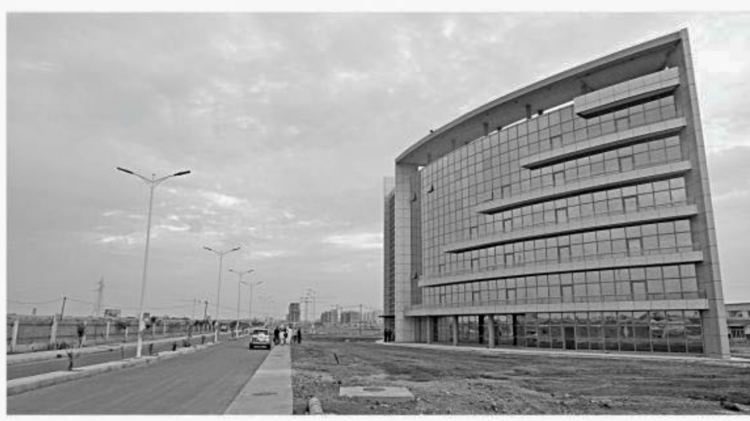
An administrative building at Senegal's new Diamniadio industrial park.
