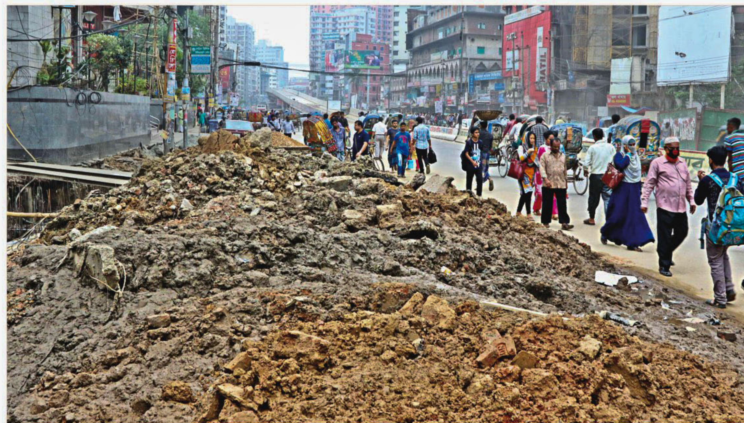
Piles of earth dug up from a road in Shantinagar to improve the drainage system. Similar development works go on across Dhaka city all the year round, only reinforcing the speculation that the capital's sewerage system has major structural flaws. This is not only putting an economic burden on the government, but also is causing public sufferings. The photo was taken near Karnaphuli Garden City. PHOTO: ANISUR RAHMAN
