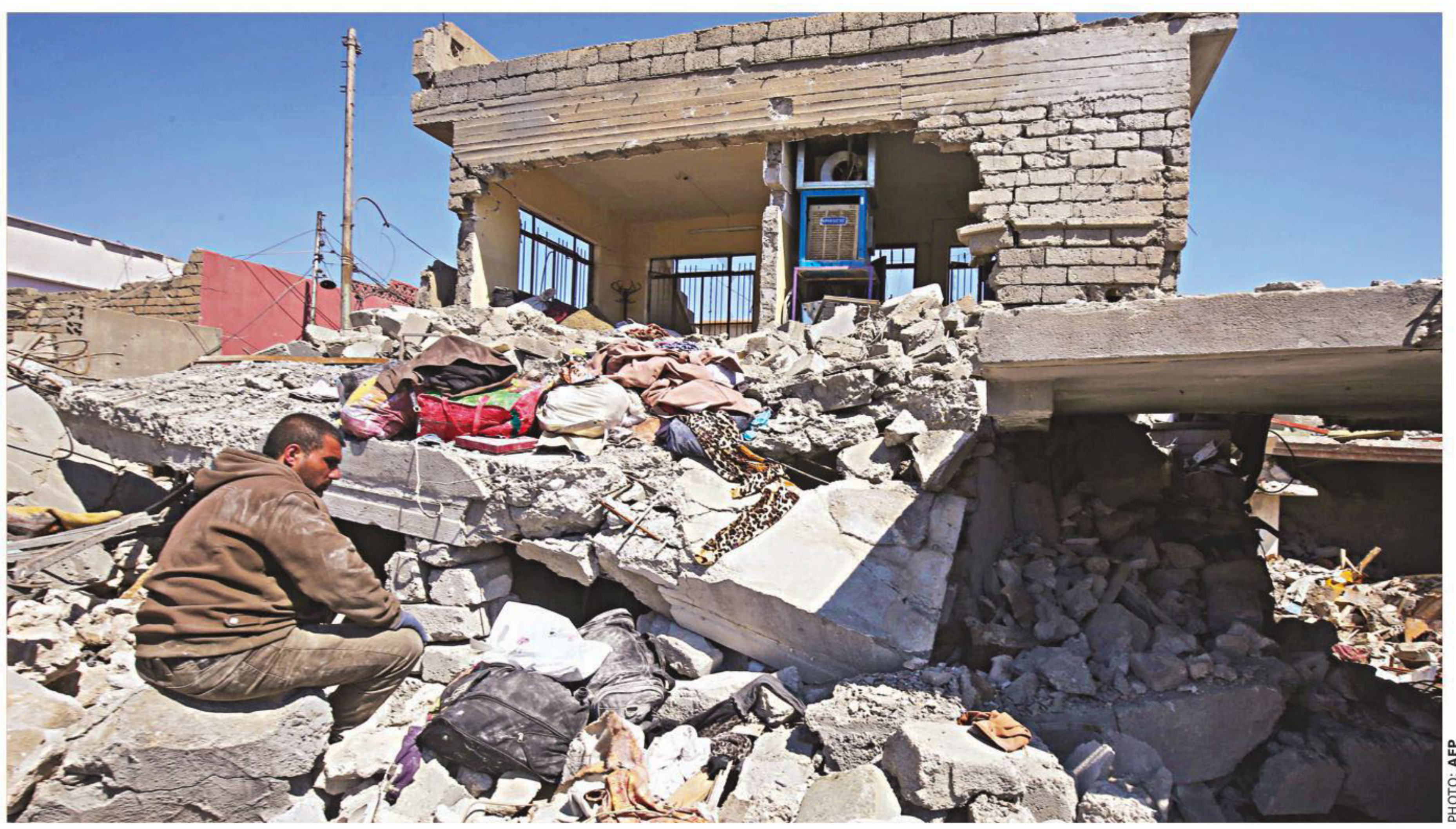
An Iraqi man sits amid the rubble of destroyed houses in Mosul's al-Jadida area yesterday, following air strikes in which civilians have been reportedly killed during an ongoing offensive against the Islamic State (IS) group. Iraq is investigating air strikes in west Mosul that reportedly killed more than 200 civilians in recent days, a military spokesman said.
