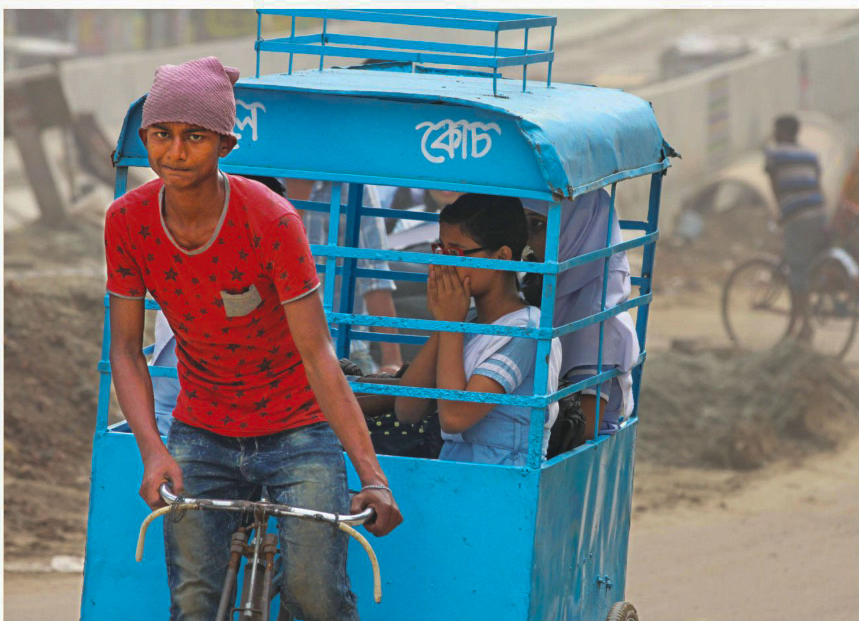
Schoolchildren cover their noses inside a school van as a cloud of dust shrouds the road near Malibagh Level Crossing in the capital around 2:00pm yesterday. The dust problem is getting worse by the day thanks to the construction of a flyover in the area, further contributing to the city's air pollution.
