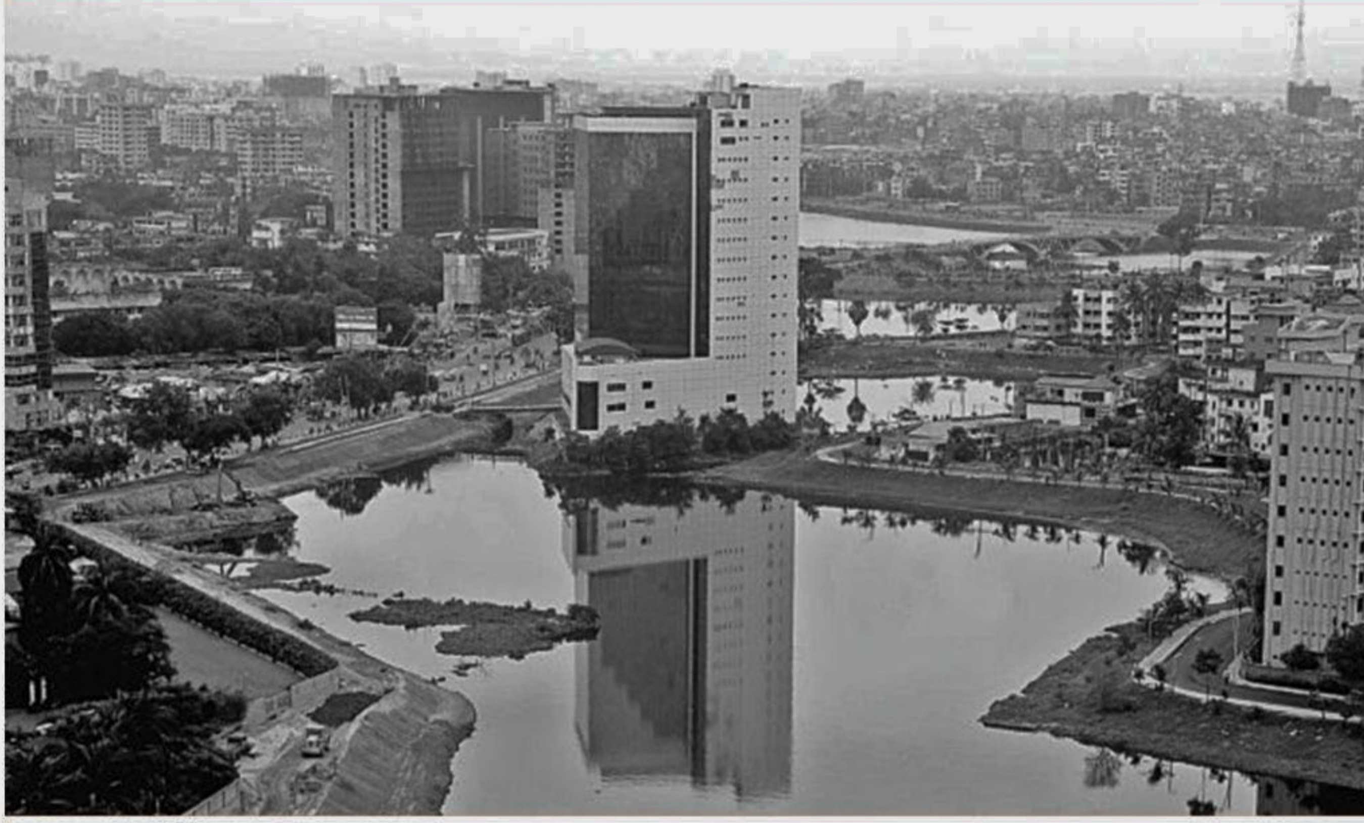
The BGMEA building in the capital's Hatirjheel awaits demolition
