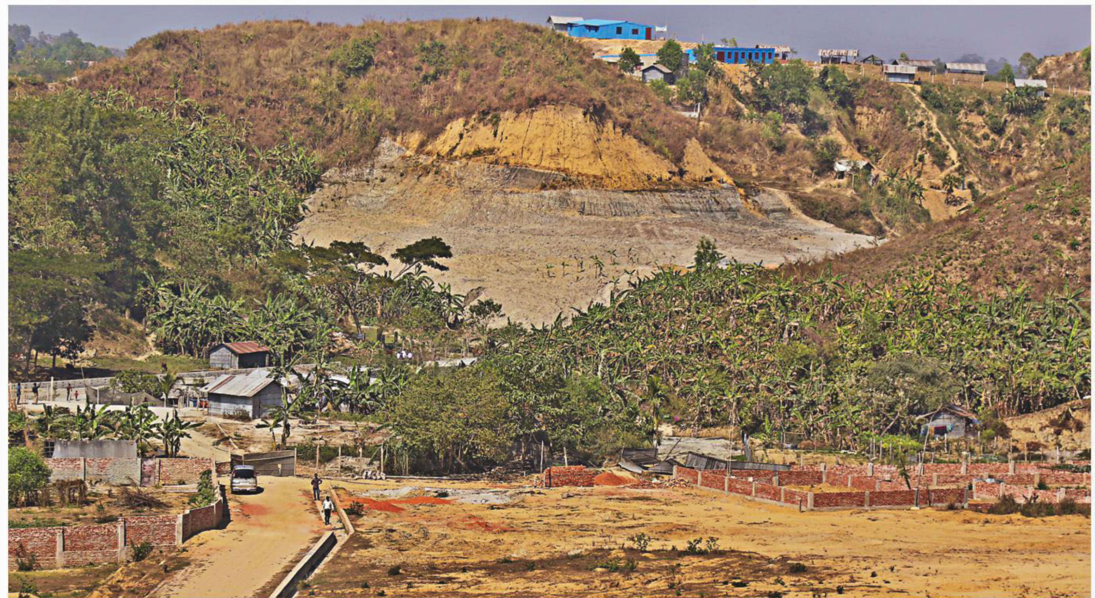
A part of the newly razed hills in the port city's Pahartali area near a housing project of Chittagong City Corporation. Illegal hill cutting continues to thrive in the area, as per locals, under the patronage of influential people. The photo was taken recently.
