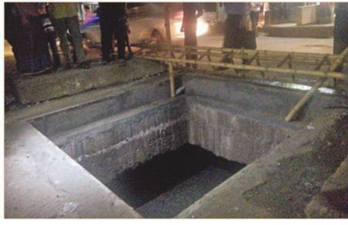
The uncovered box culvert in the capital's Paltan area.
