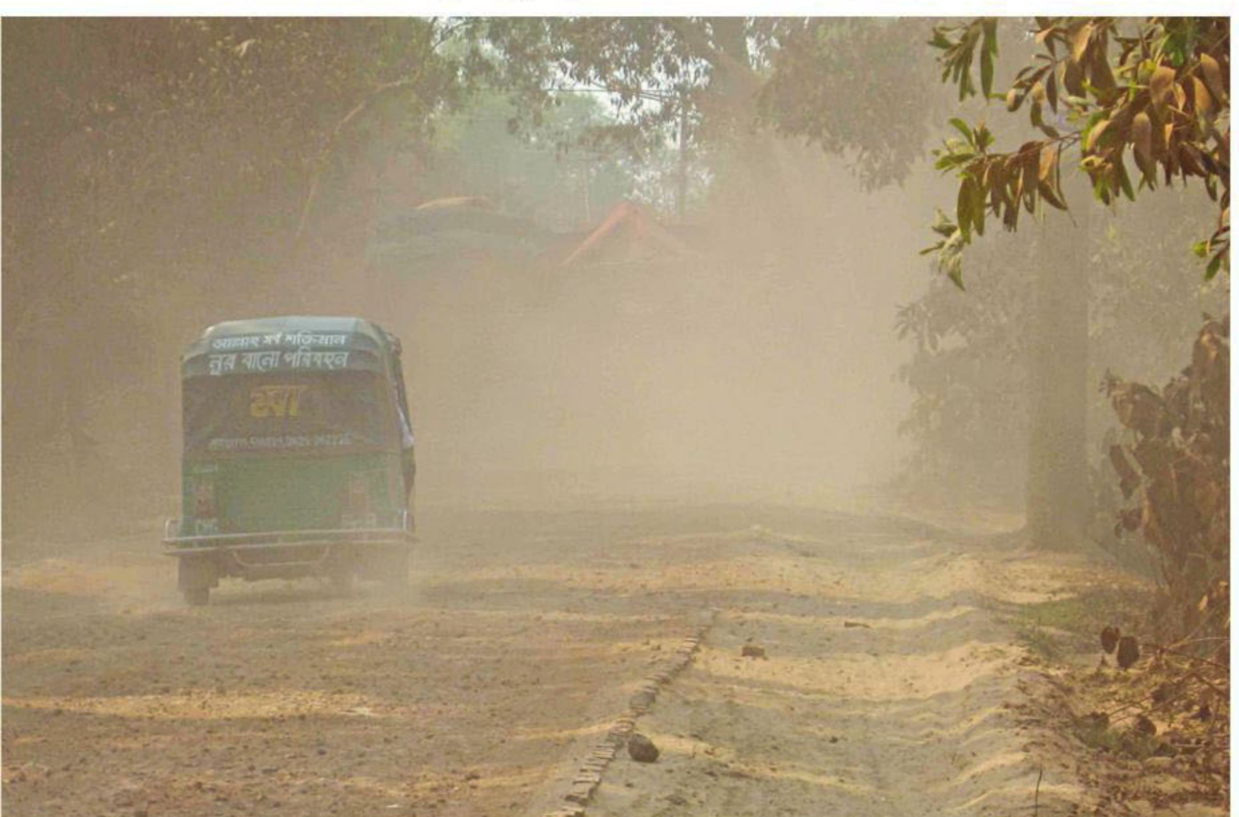
Thick cloud of dust from this incomplete road makes it almost impossible to see even the largest vehicle only a few feet away. The five-kilometre stretch of the road, connecting Gararon and Bormi Bazar in Gazipur, has been in a deplorable state for nearly three years. The condition worsened eight months back when the authorities laid brick rubble as bottom layer on the road as part of a repair project. The unfinished work left the brick rubble exposed, causing the formation of dust when vehicles ply the road. Crops and trees in the area are now covered with reddish brick dust. Residents in the area are the worst sufferers as many of them now have respiratory complications. The photo was taken recently.
