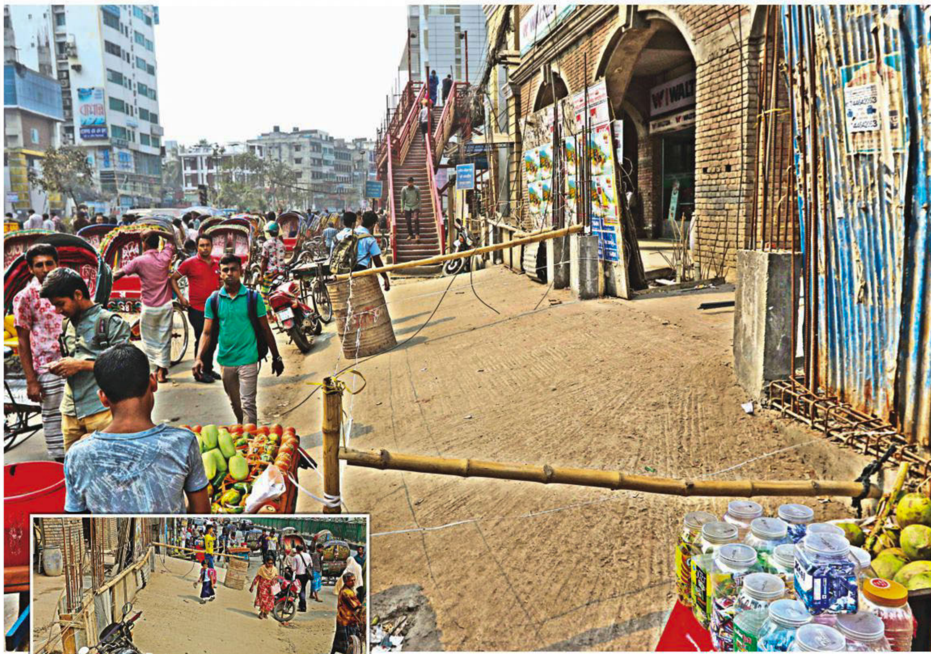
WHOSE FOOTPATH IS IT ANYWAY? A ramp has been built on part of the footpath to facilitate the exit and entry of cars at the gate of a building near the capital's Bangla Motor intersection. The photo was taken yesterday. PHOTO: ANISUR RAHMAN
