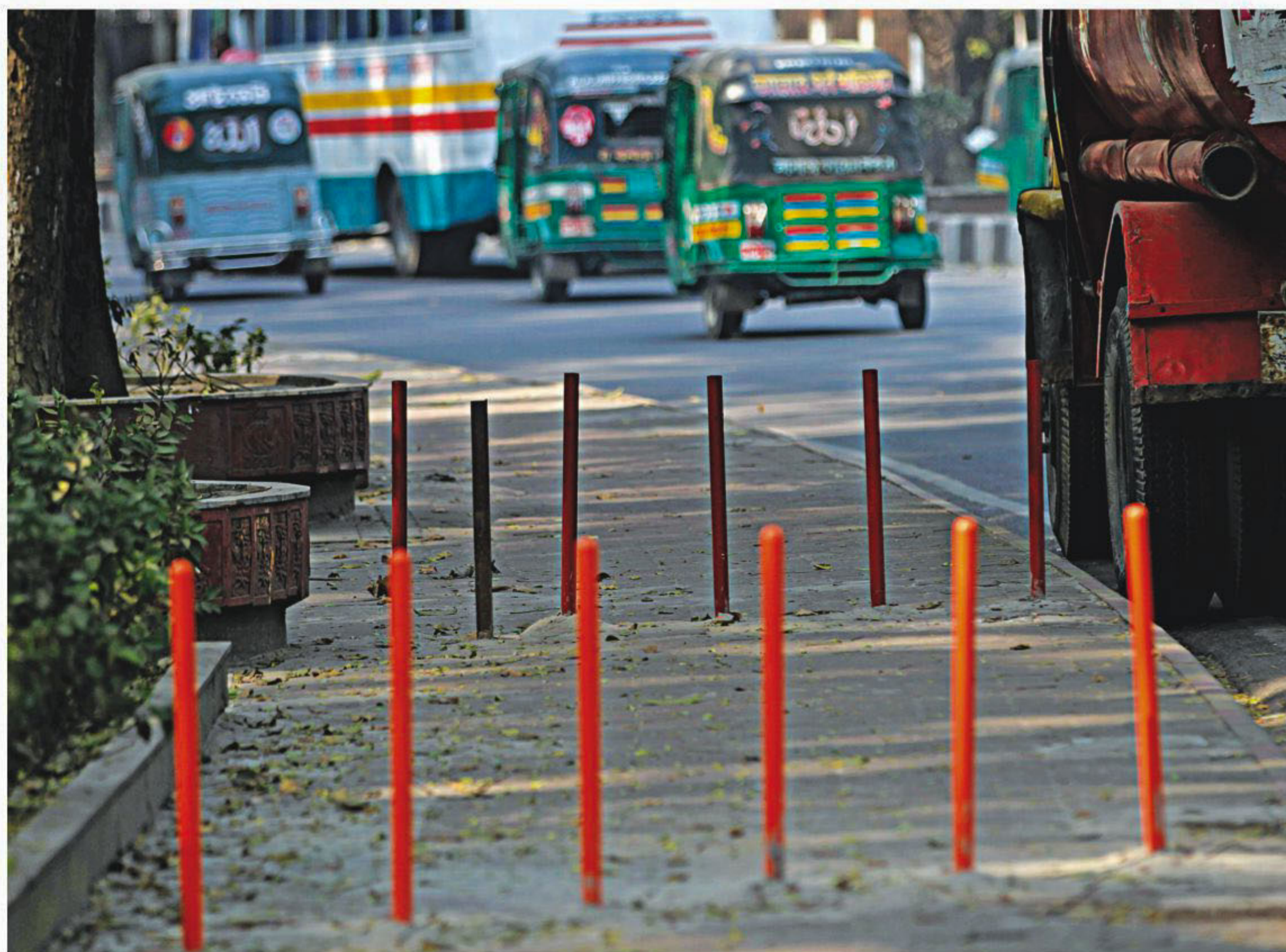
Iron rods have been installed on the pavement in two rows on Hare Road in the capital so that motorbikes cannot use the pavement. The photo was taken yesterday near Ramna Park.
