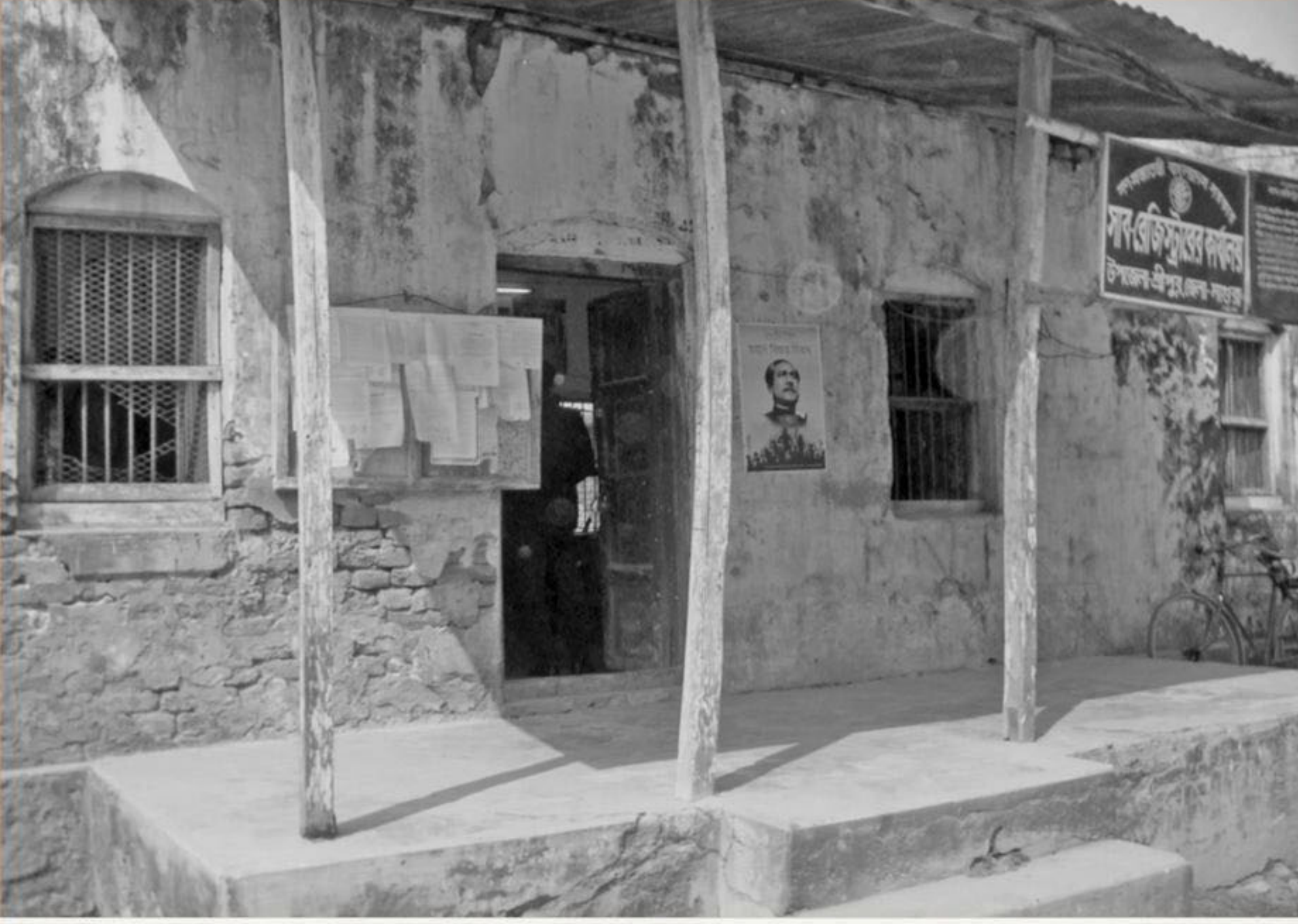
The dilapidated Sreepur sub-registrar's office in Magura.
