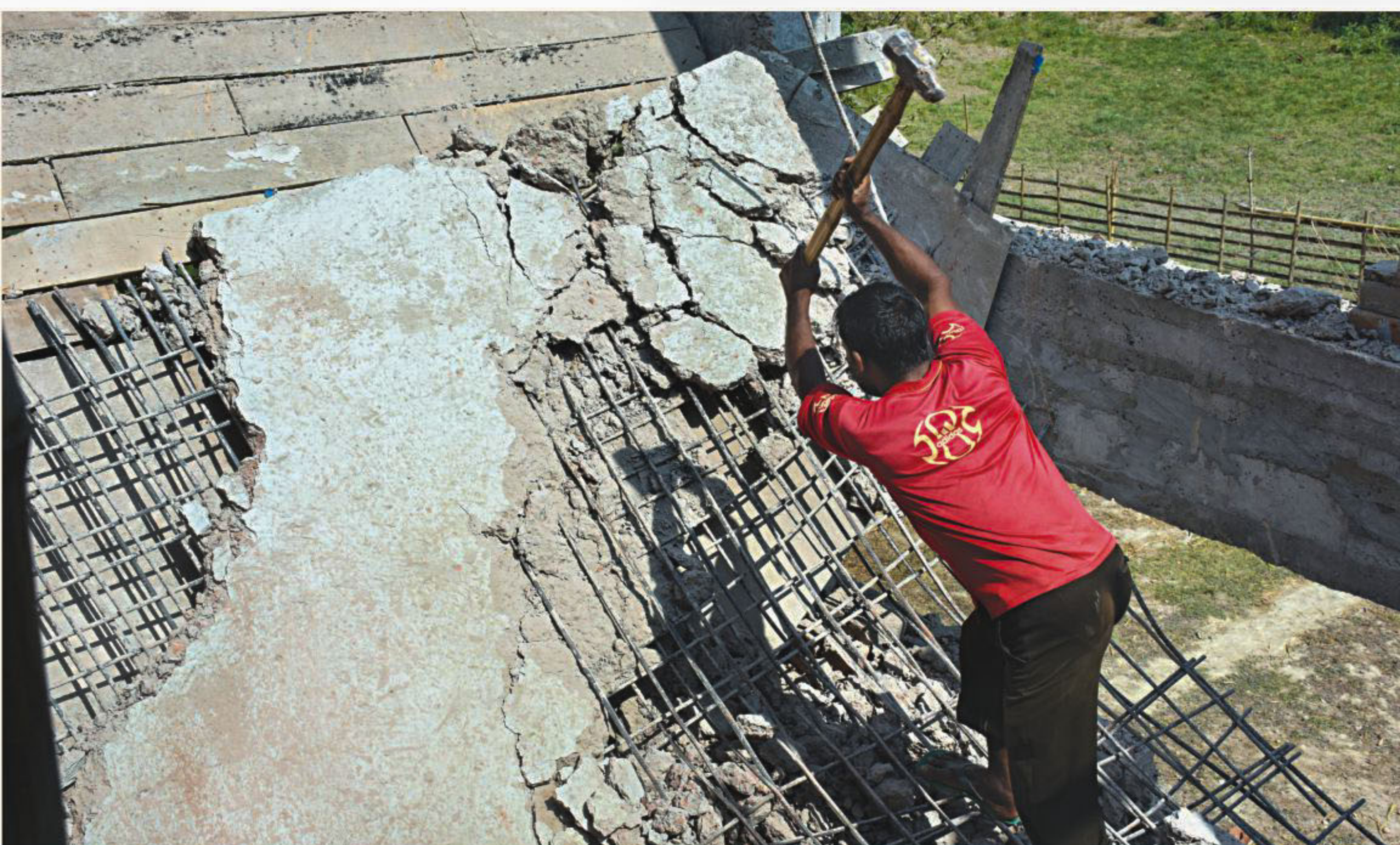
A worker demolishes the under-construction two-storey building of Nabinpur Government Primary School in Meherpur's Gangni upazila yesterday. The LGED office in Meherpur asked the project contractor to knock down the building as it was built with low-quality materials. The contractor will rebuild the school.
