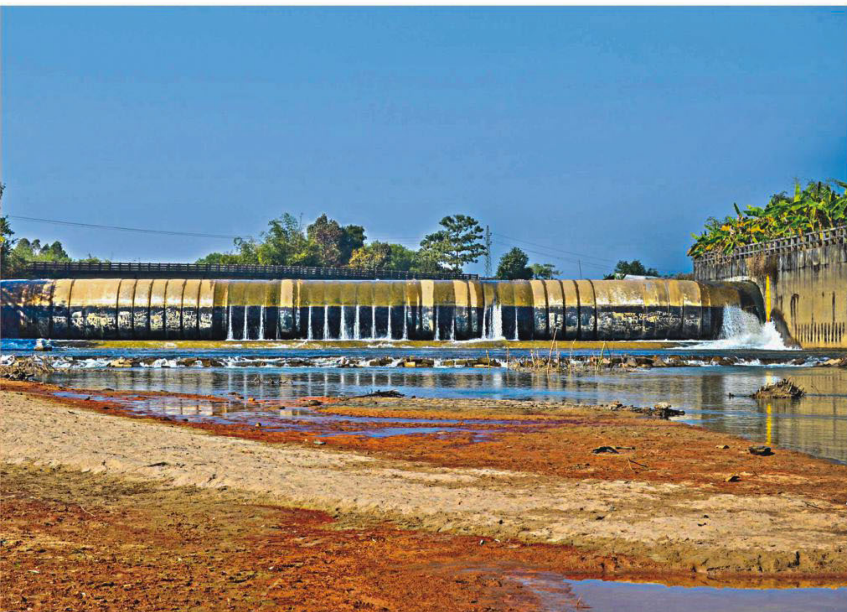
A rubber dam on the upstream of the Halda disrupting its natural flow. The photo was taken recently.
