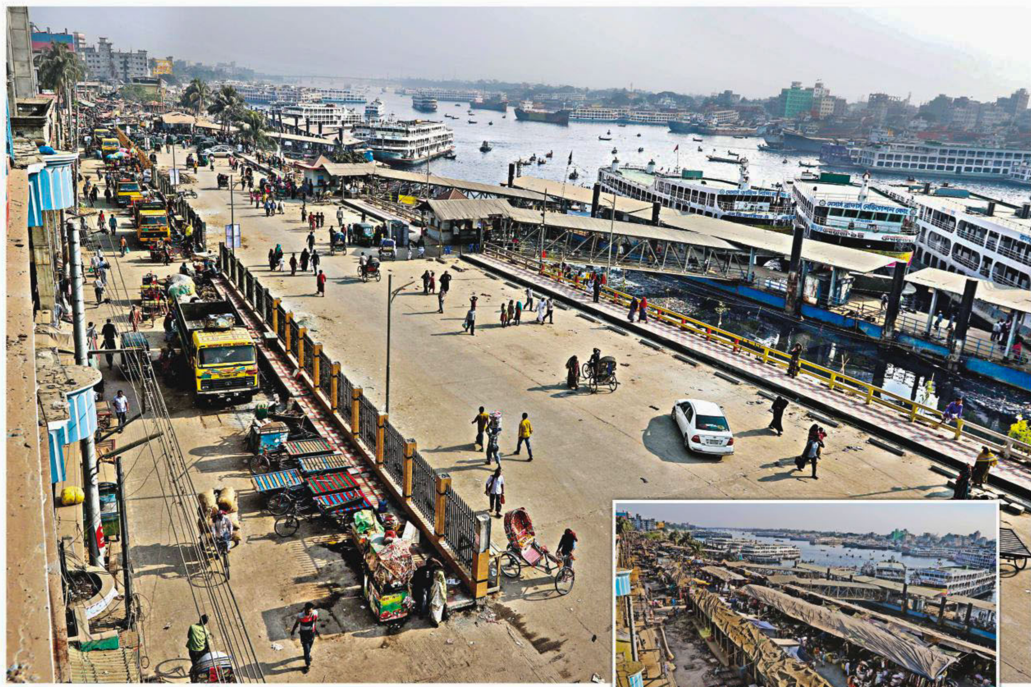
Illegal shops built on the Buriganga river bank between Sadarghat and Shyambazar in the capital are now gone following steps by the BIWTA. Inset, the illegal shops were occupying the place a few days ago.
