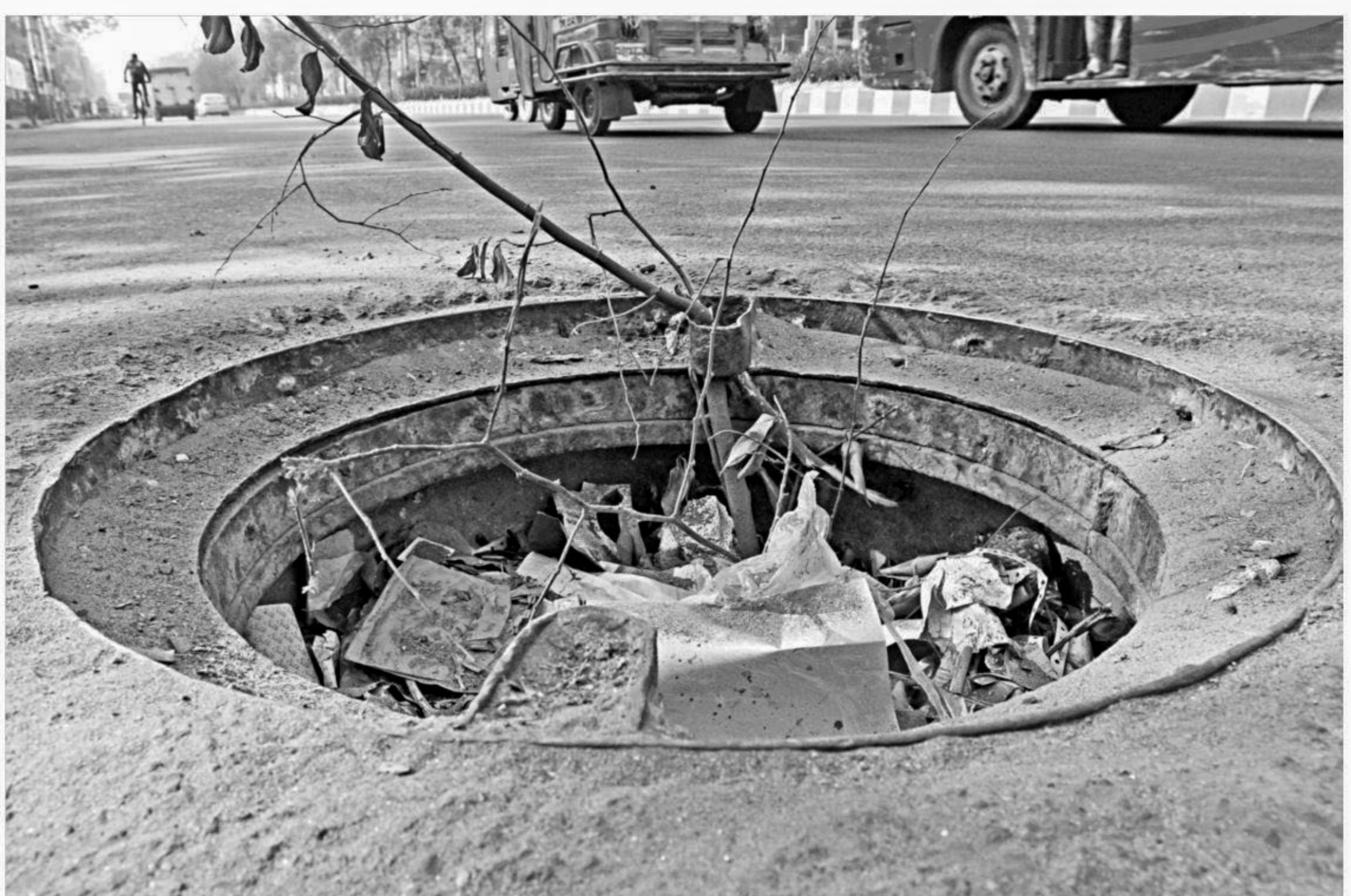
Dried up branches of a tree juts out of a lidless service manhole on a road in the capital's Tejgaon Industrial Area as a warning to approaching vehicles. With none bothering to rectify the situation, the hole has become a waste destination clogging the sewerage line and contributing to the area's waterlogging. The photo was taken yesterday morning. PHOTO: SK ENAMUL HAQ
