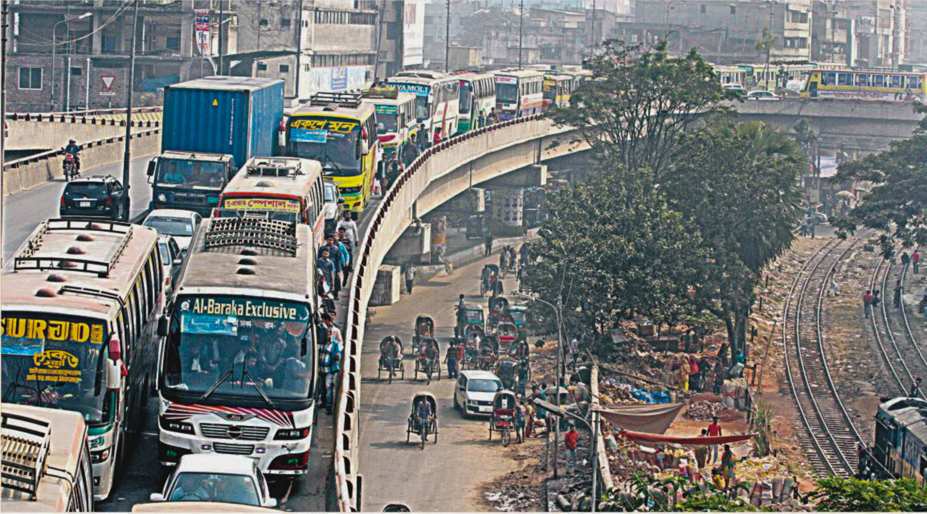
Numerous vehicles clog the capital's Khilgaon flyover while trying to avoid the Malibagh level crossing-Rampura road, which is being renovated. The photo was taken around noon yesterday. PHOTO: SK ENAMUL HAQ
