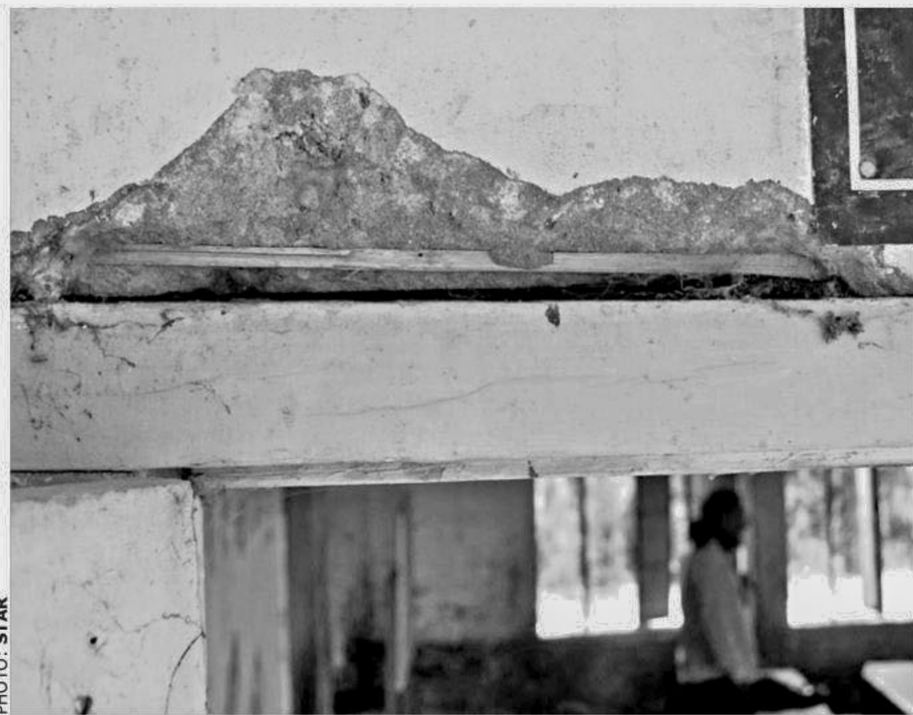
KIDS UNDER RISK, WHO CARES: Chunks of plaster fall off, revealing the bamboo sticks that were used instead of iron rods to construct the building of Binnadangi Government Primary School in Pabna and right, bamboo poles are set to support the weakened concrete beam at a classroom of Chapali Government Primary School in Jhenidah.
