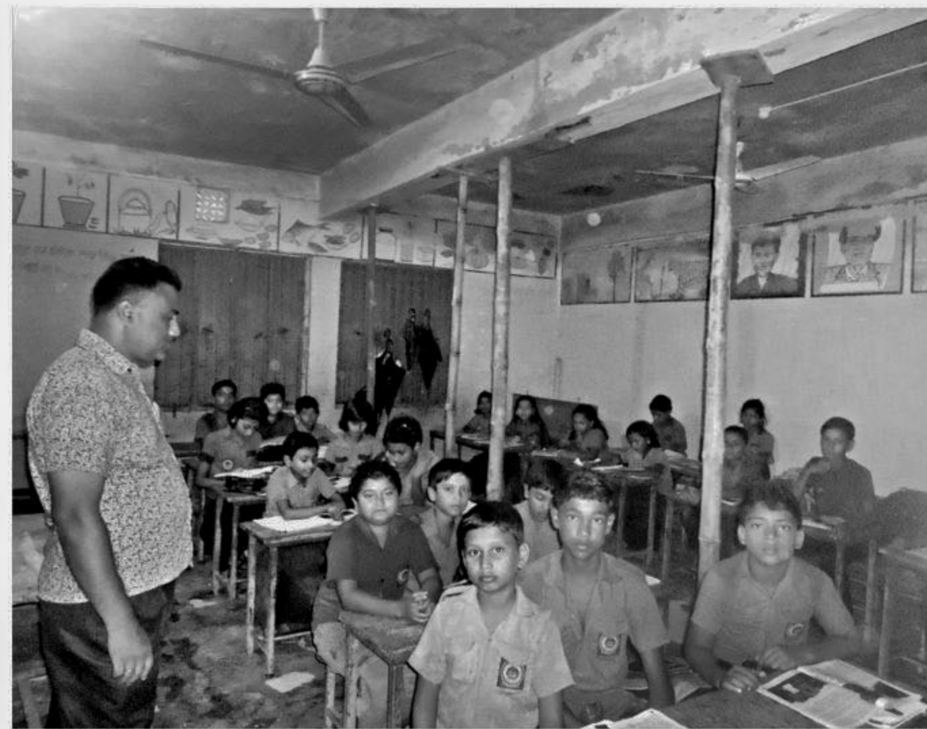
KIDS UNDER RISK, WHO CARES: Chunks of plaster fall off, revealing the bamboo sticks that were used instead of iron rods to construct the building of Binnadangi Government Primary School in Pabna and right, bamboo poles are set to support the weakened concrete beam at a classroom of Chapali Government Primary School in Jhenidah.
